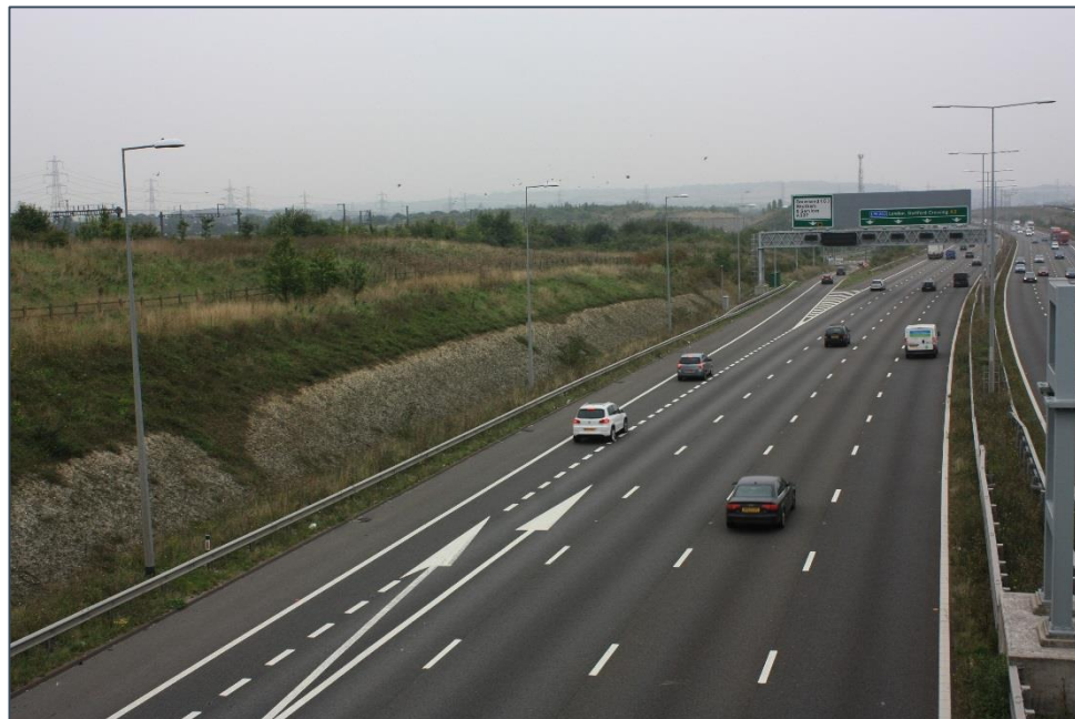
Figure 5.6 Chalk Cutting Slopes on A2 Showing Colonisation with Wildflower Grassland Above
