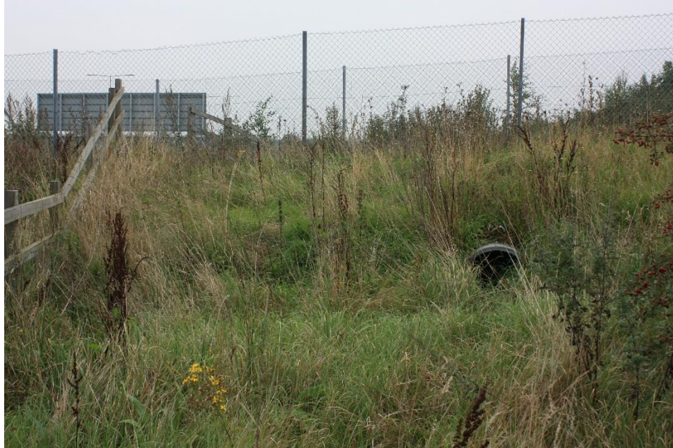
Figure 5.7 Badger Tunnel Adjacent to the Ifield Court Overbridge
