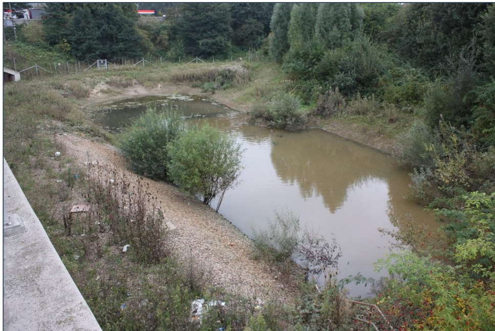
Figure 5.10 Infiltration Pond at Cobham Services
