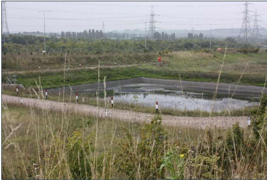
Figure 5.8 Attenuation Pond B at Downs Road
