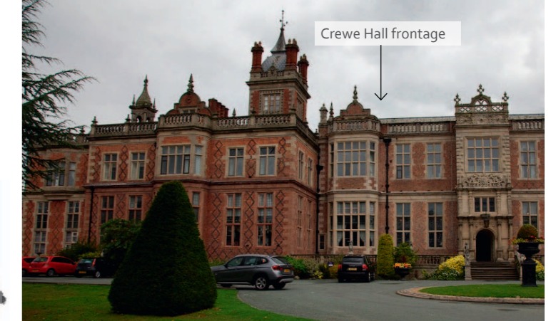
Figure 2: Crewe Hall frontage, from the southern approach
