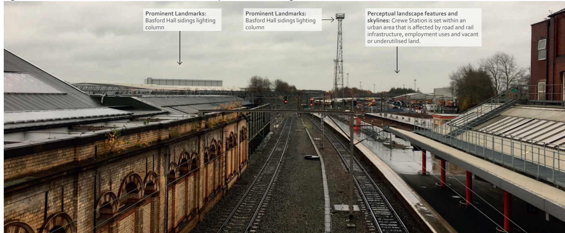
Figure 4: Crewe Station and WCML rail infrastructure from pedestrian overbridge
