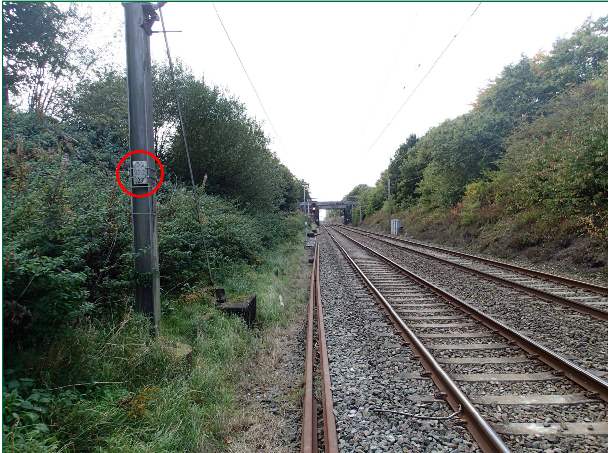
Figure 2: Location of the accident as viewed in the direction of travel of train 1F22 on the approach to HN103 signal, visible in the centre of the picture, and the OLE mast identification plate (ringed)
