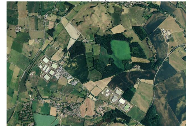
Hopton village below with MoD bases and enclosed Hopton Heath and registered battlefield site above.
