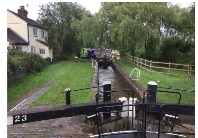
Hoo Mill Lock and lock keeper's cottage on the Trent and Mersey canal. Looking north.
