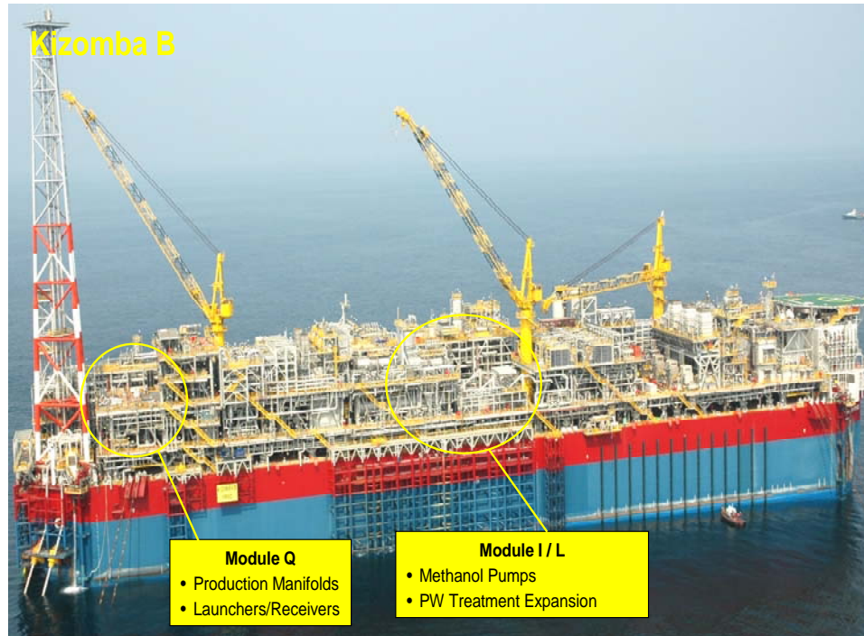
FIGURE 4-10: Kizomba B FPSO Topsides Modifications
