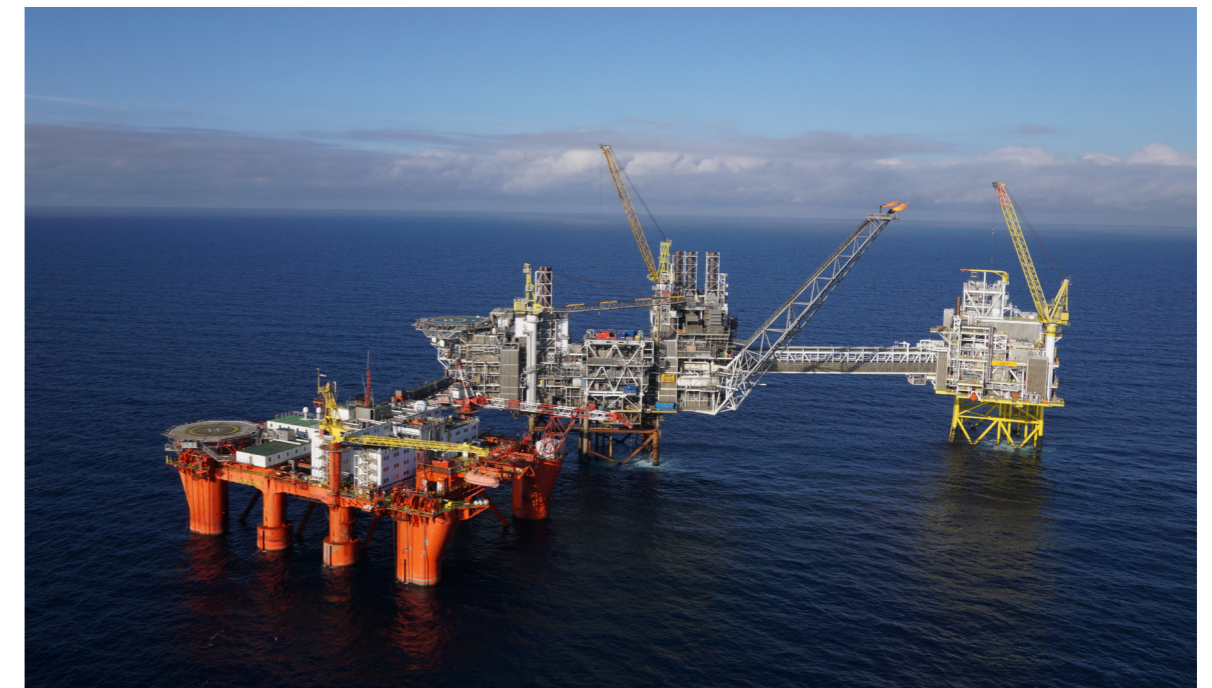
The COSL Rival mobile accommodation unit at the Judy Platform.
