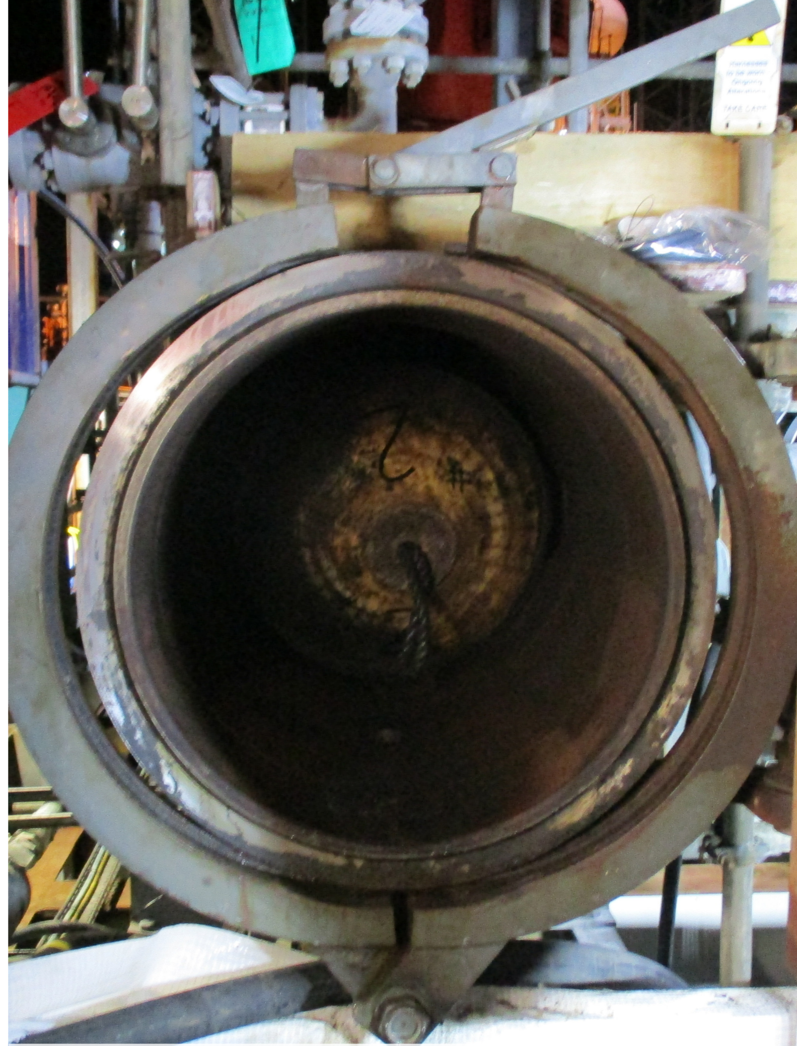
Launching a pig during the flushing of the Viking export pipelines.
