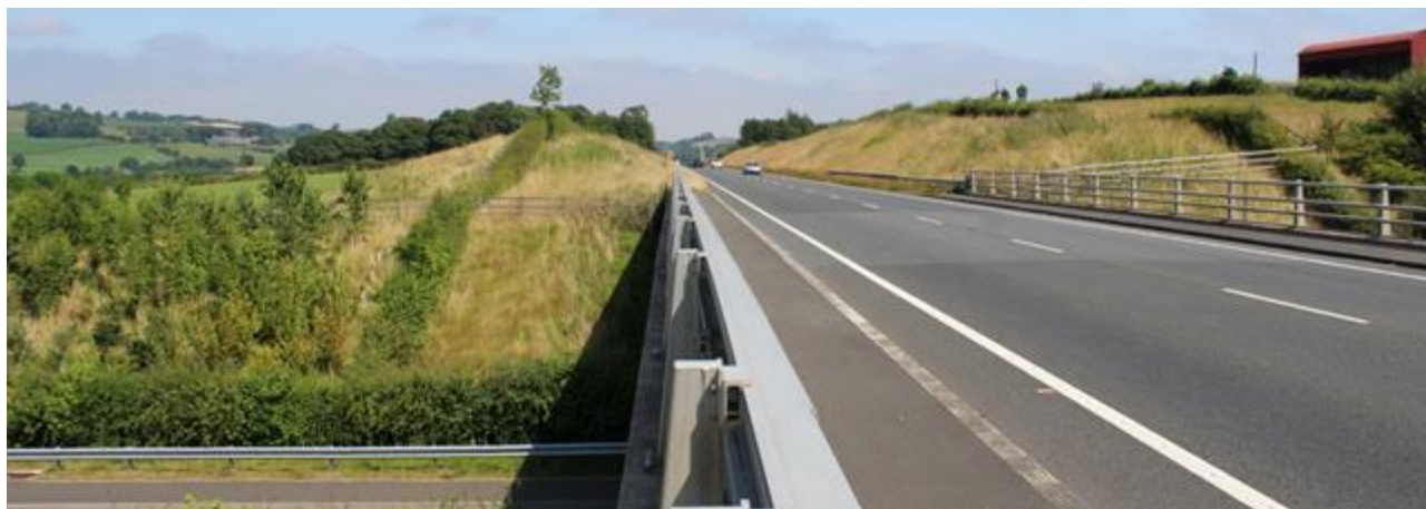
Figure 5.2 Example of noise mitigation earthworks view east along bypass at Cemetery Road Bridge - false cutting on left with hedge along crest and cutting slope on right
