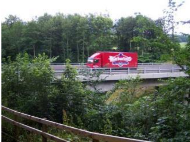
Figure 9.11 OYA Gees Wood looking south towards bypass bridge
