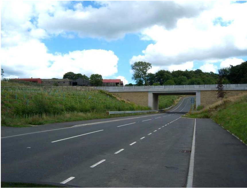
Figure 9.21 OYA Bridge Crossing Cemetery Road
