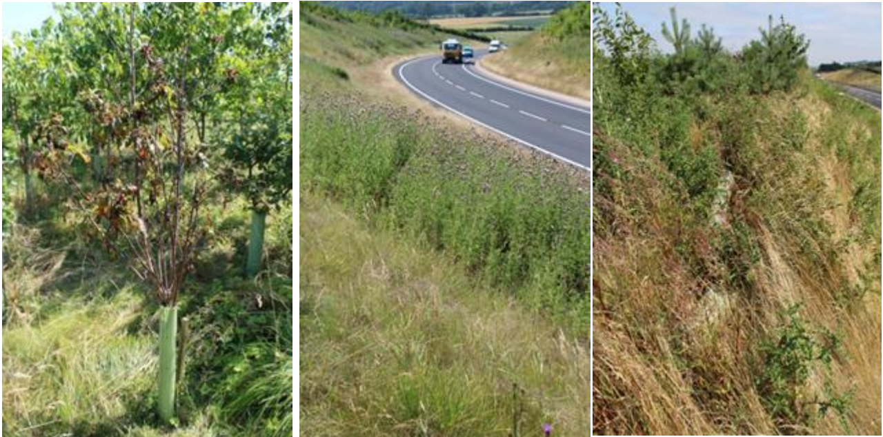
Figure 5.9 Lack of recent maintenance within planting plots (right)
