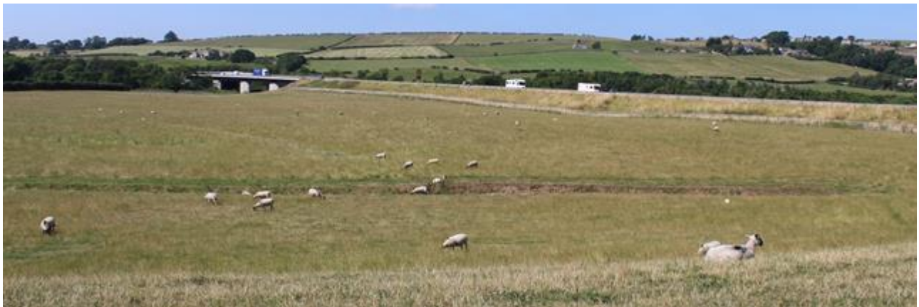
Figure 5.11 Looking towards bypass from East Land Ends Lane across area restored to agricultural use
