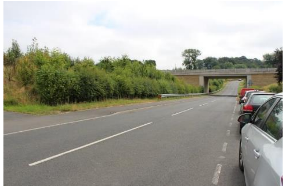
Figure 9.22 FYA view – hedge and woodland planting has established well. Hedgerows were expected to act as bat flight lines under the bridge.
