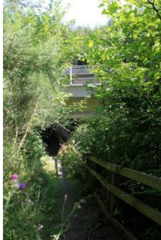
Figure 9.12 FYA from similar point on the footpath demonstrating good regrowth of adjacent vegetation
