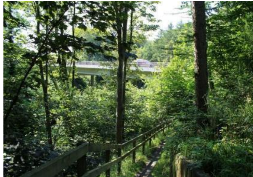
Figure 9.14 The FYA view - Scrub planting was intended to act as a long term flight path for bats encouraging them to fly under the bridge and away from vehicles on A69. ES plans indicate that scrub should be managed to draw bats under not over the bridge
