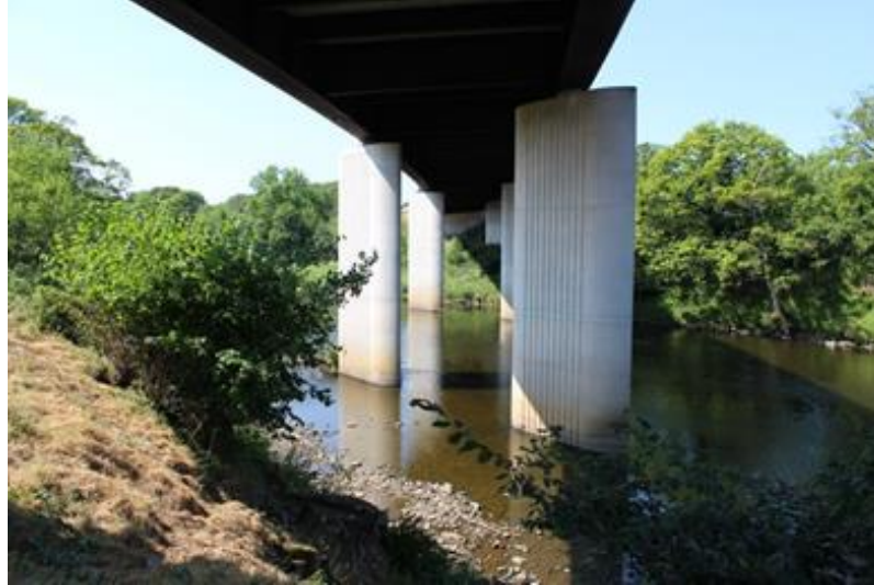
Figure 5.25 Haydon viaduct – new bridge crossing of the River South Tyne
