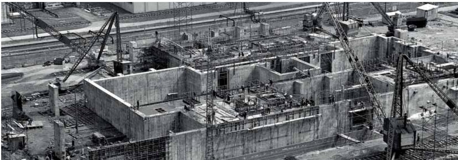
The pond under construction in 1958
