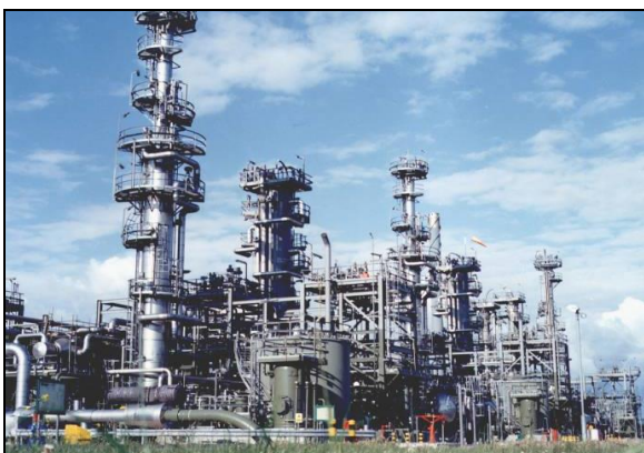
Photo 5 - POA Gas Terminal
