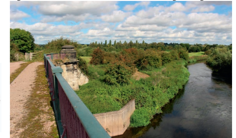
Figure 3: View to the north from historic High Bridge
