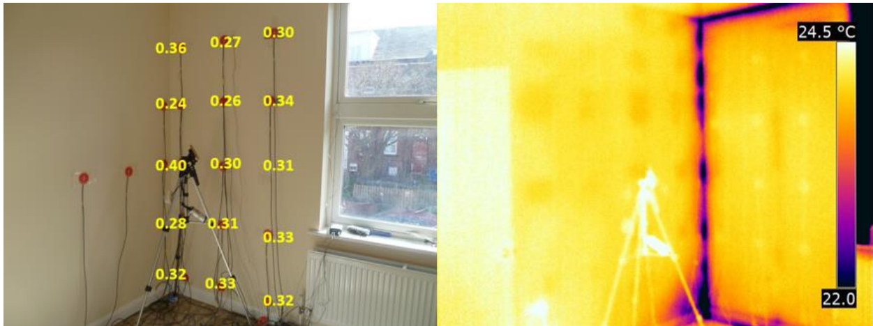
Figure 6: Annotated image and thermogram showing the post-retrofit external wall U-value measurements
