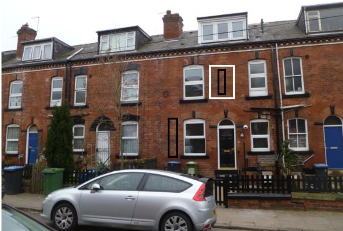
Figure 2: Area of external wall subject to U-value measurements (black regions – pre-retrofit, white region – post-retrofit)
