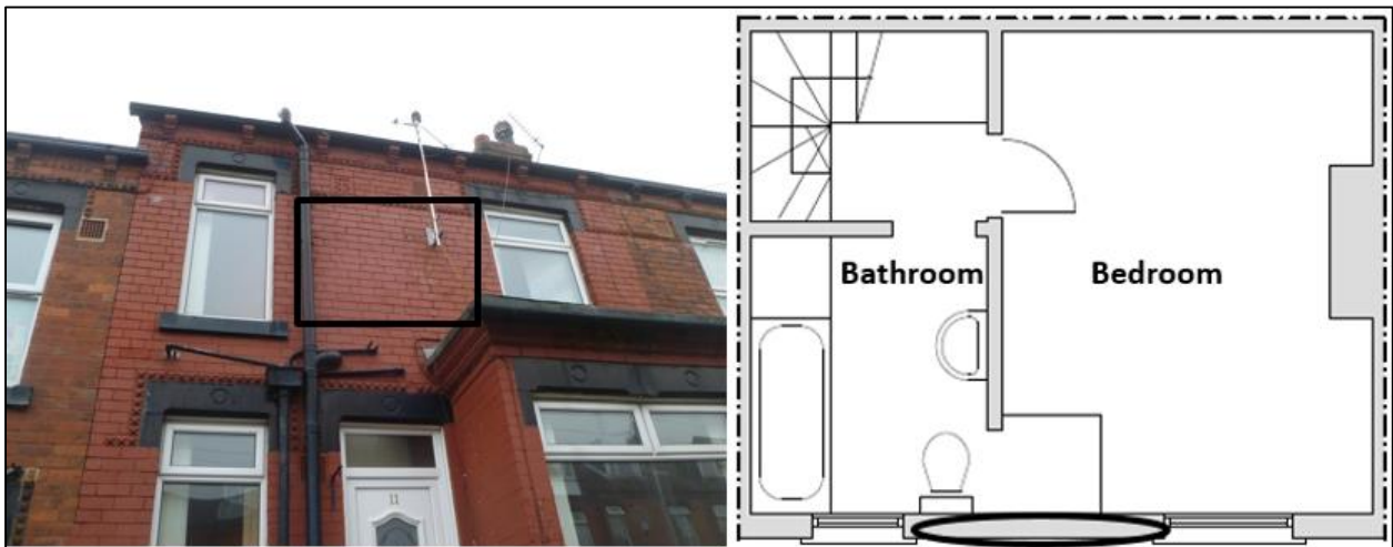
Figure 3: Area of external wall subject to U-value measurements (marked in black)
