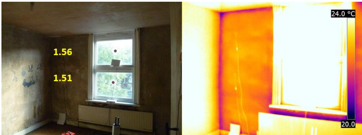
Figure 4: Annotated image and thermogram showing the first floor pre-retrofit external wall U-value measurements
