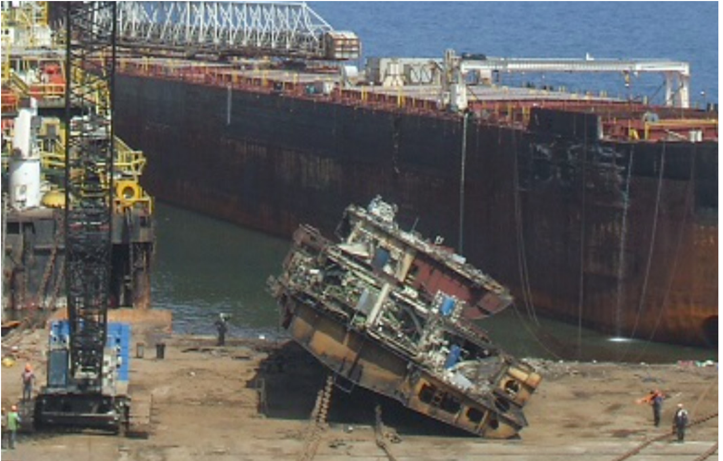
6 Aug 2016 - Demolition works nearing completion.
