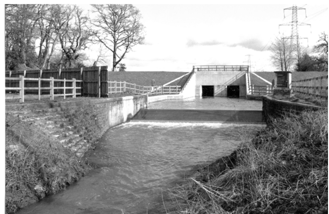
Flood alleviation downstream of Yate is provided by Tubbs Bottom flood storage area – photo to right shows the outlet structure
