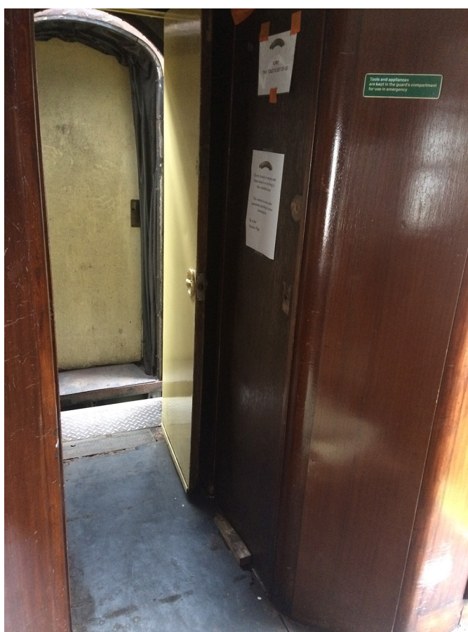
Figure 4: The outside of the toilet cubicle involved in the accident
