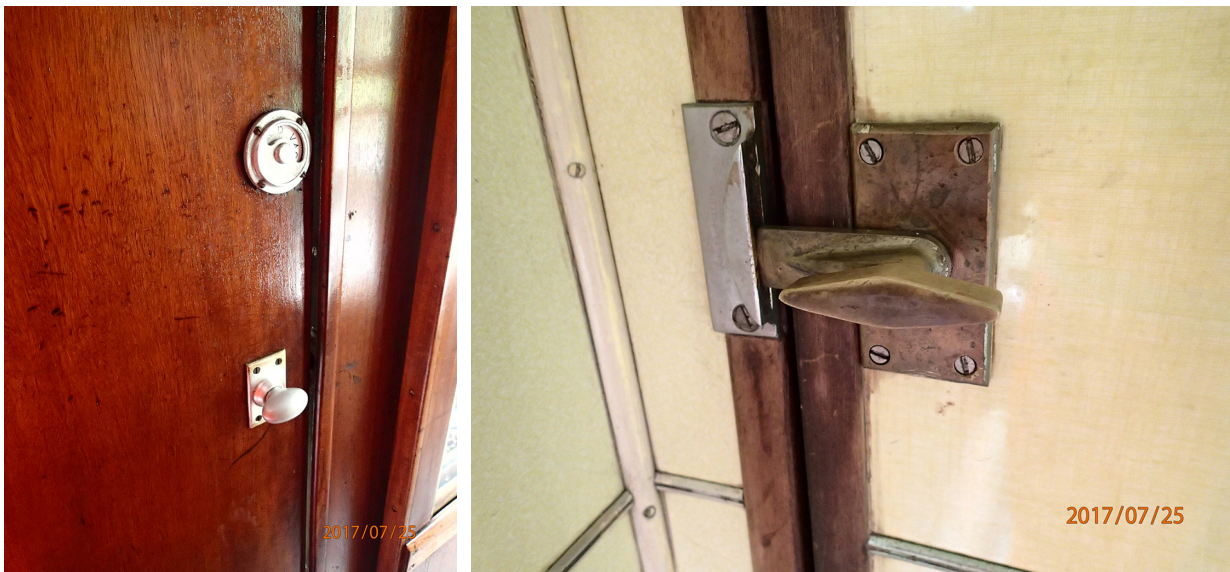
Figures 6 and 7: Typical layout of a door locking arrangements on a toilet cubicle on a British Rail Mark I carriage
