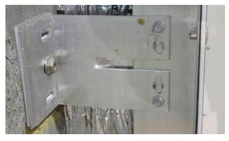
Figure 9. Example of aluminium rail fixed to 'L' bracket through fixed holes.
