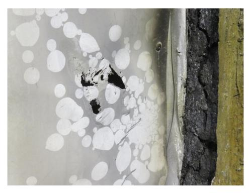
Figure 26. Close up view of partial panel consumption on the wing wall.
