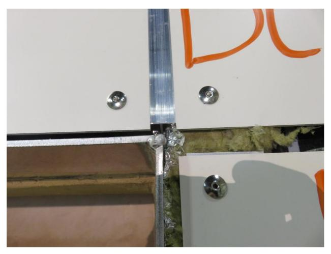
Figure 11. Detail at corner of combustion chamber opening. Panels riveted in place with nominal 20mm vertical gap for ventilation purposes.
