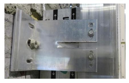
Figure 8. Example of aluminium rail fixed to 'L' bracket through movement holes.
