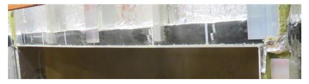
Figure 5. Horizontal intumescent cavity barriers fixed through the entire depth on face turned steel brackets, fitted above window pod.
