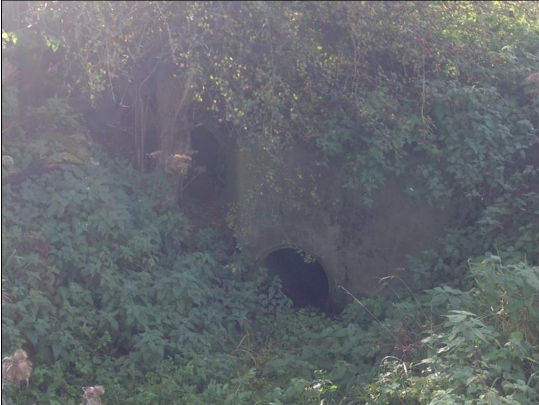
Figure 2: Inlet to culverts under Bent Lane
