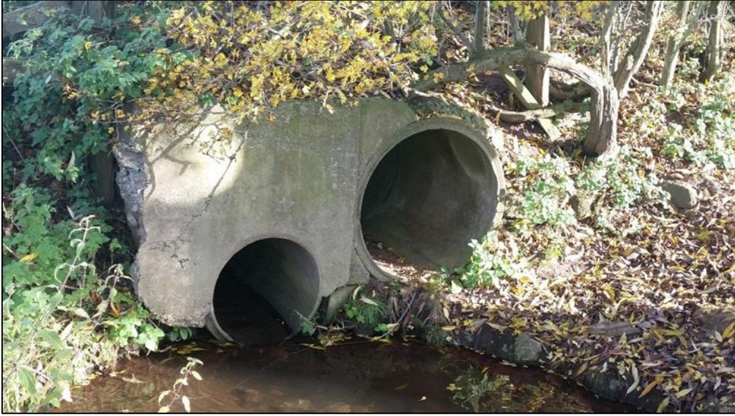
Figure 3: Outlet to culverts under Bent Lane
