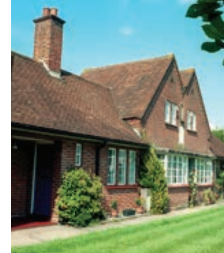
The bungalow (House 35) looked little different on the outside after the retrofit.
