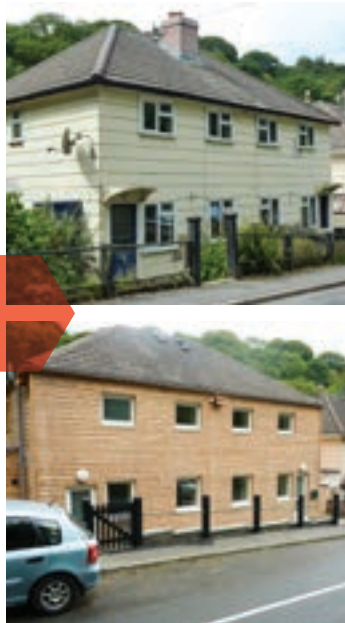
House 69 before (top) and after (bottom) the retrofit. Note the deeper window reveals (depth of cills) as a result of adding external wall insulation.
