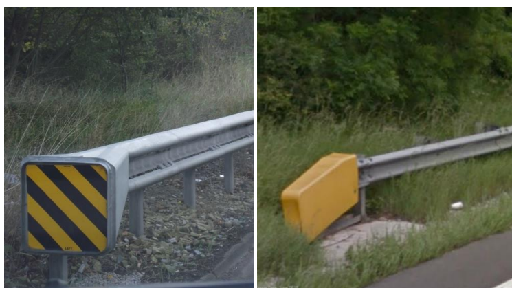
Figure A11.3 – Examples of Terminals
