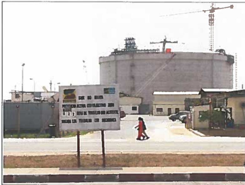
Figure 6-10: Kwanda Base in Soyo, the centre point for the oil industry in the region.
