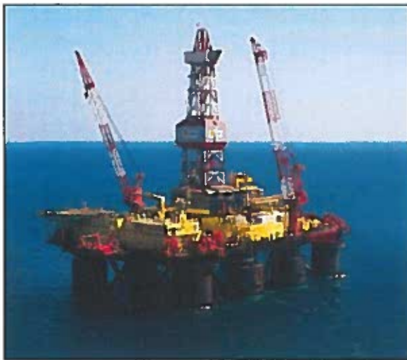
Figure 4-1: The Scarabeo 7 drilling unit.
