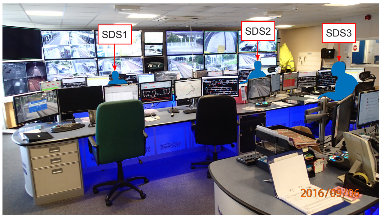
Figure 5: Control room office
