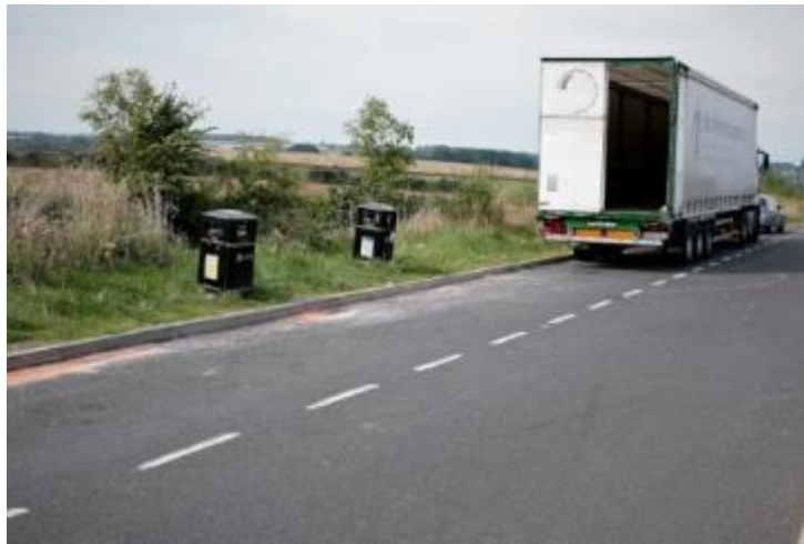
Figure 5.22 The lay-by on the northbound carriageway of the LAR between Wattle Syke and Wetherby
