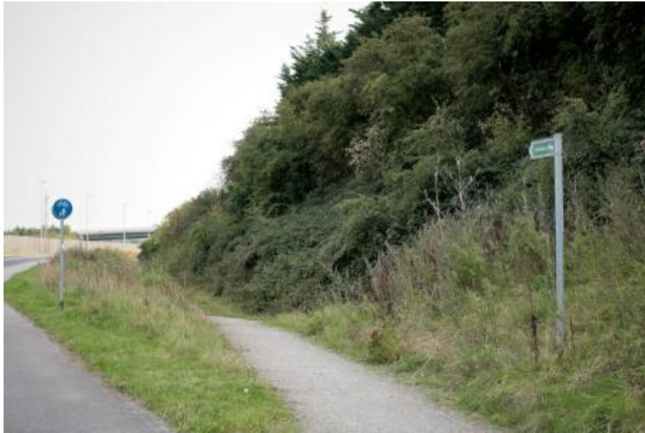
Figure H.12 Privas Way: additional NMU signage has been provided
