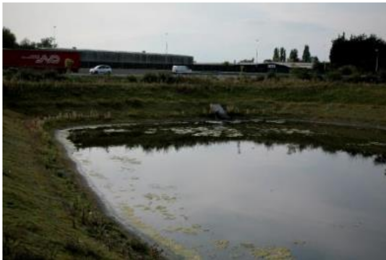
Figure 5.18 Sandbeck Balancing Pond
