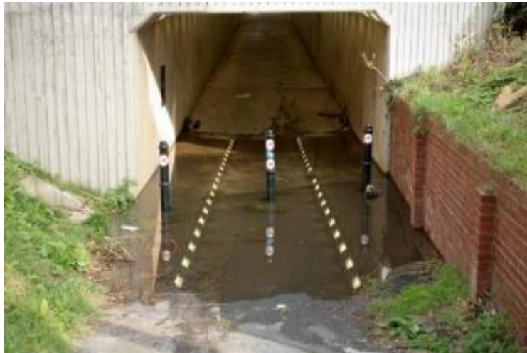
Figure 5.13 Ponding at the western end of the Freemans Way underpass, adjacent to the LAR
