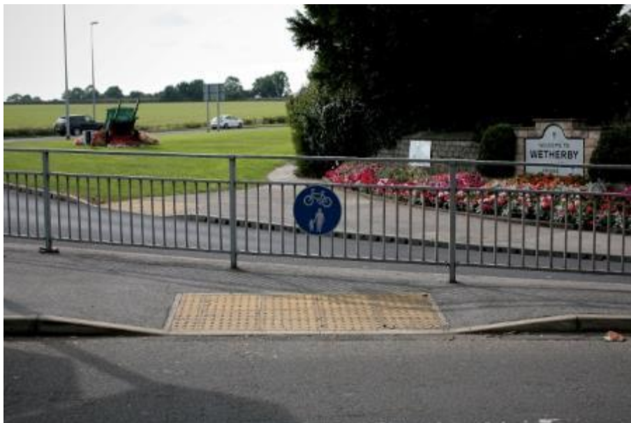
Figure H.6 Splitter island with shared use sign installed on railings
