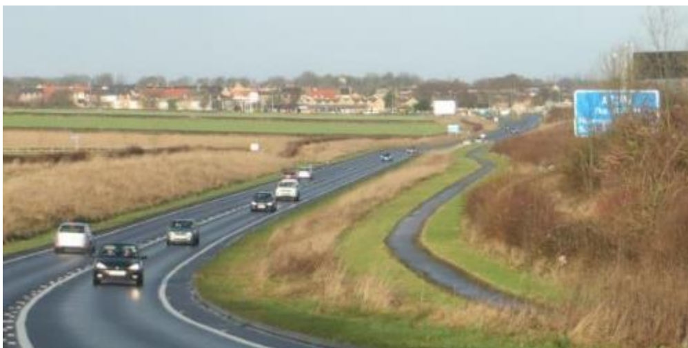
Figure 6.1 NMU Facility between the LAR (left) and A1(M) (obscured to the right)
