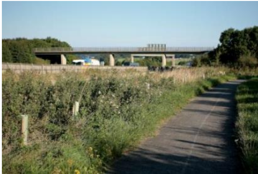
Figure 5.8 Notable areas where planting is not as vigorous as perhaps would be expected are along the NMU route adjacent to the southbound carriageway of the A1(M) south east of the Paradise Farm overbridge (top) and adjacent to the southbound carriageway of the A1(M) north of Walton Road overbridge (bottom)
