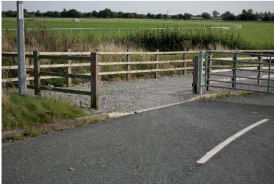
Figure H.8 A drop crossing has been provided for NMUs at York Road
