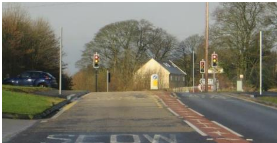
Figure 3.7 Junction of Paradise Way for Bramham Park on the LAR
