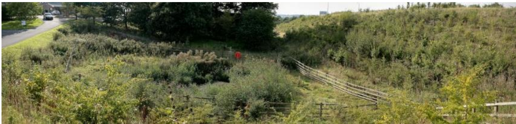
Figure E.6 Park Hill Farm Ecological Pond at FYA (September 2014)
