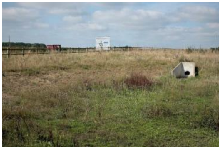
Figure 5.19 Wattle Syke Infiltration Pond
