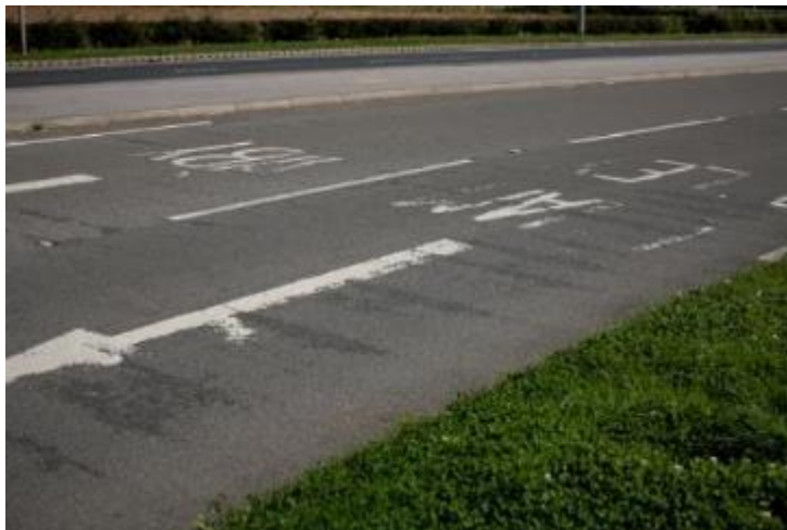
Figure 5.23 Typical examples of the faded road markings at the Wattle Syke roundabout; approaching the roundabout (top) and on the roundabout (bottom)
