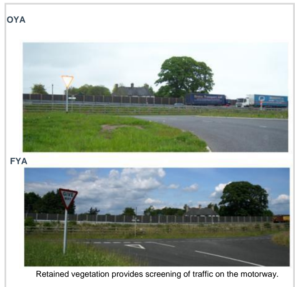
Figure 9.21 OYA and FYA acoustic barrier at Mossband
