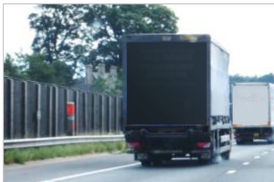
Figure 3.5 FYA: emergency phones on the M6 J44 - 45
