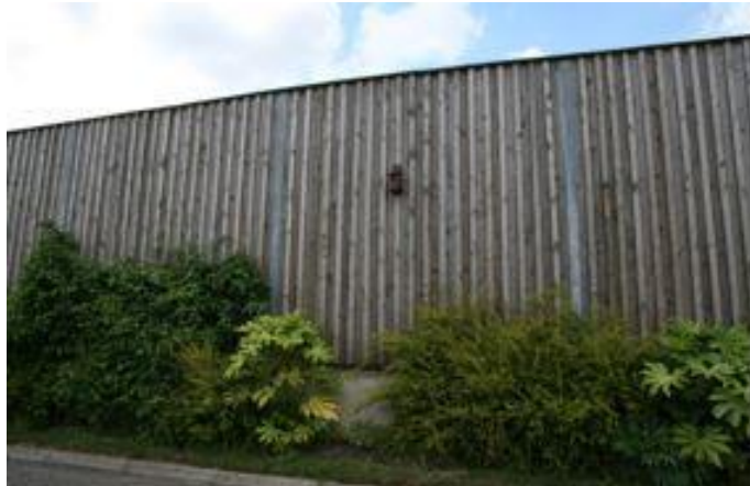
Bird boxes attached to environmental barrier and screening plating
