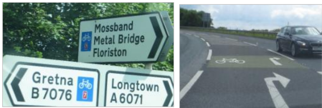
Figure 6.2 Signing and Lining supporting Route 7
