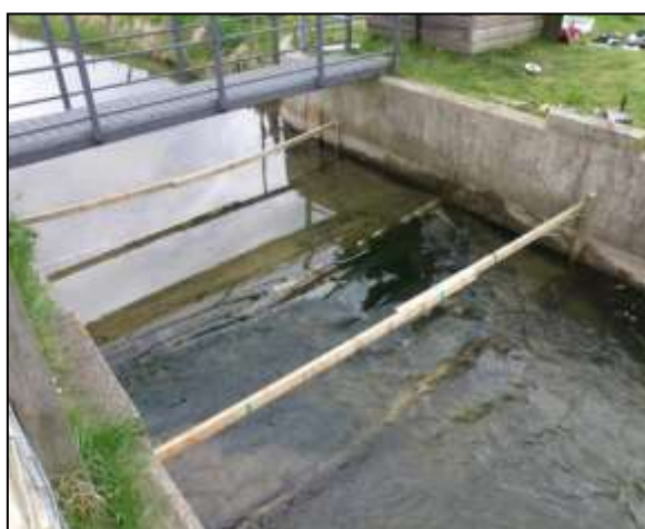
Figure 7.1 PIT telemetry configurations installed at 2 flow gauging weirs to track eel passage
