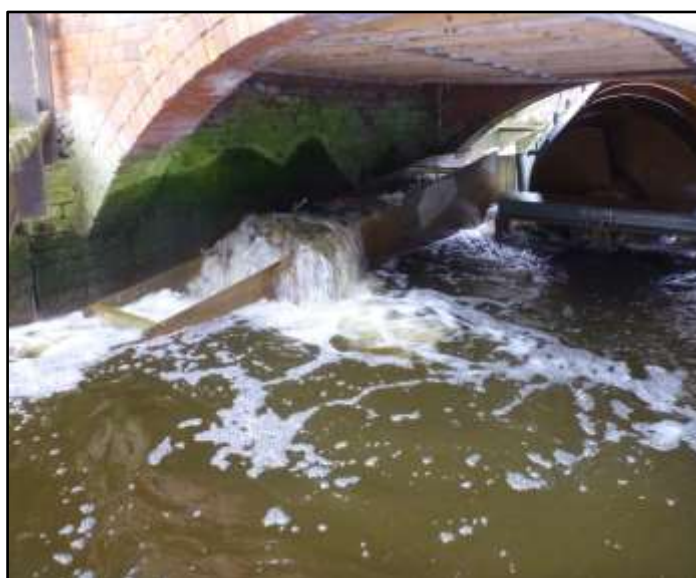
Figure 4.2 Woody debris and vegetation causing partial blockage in the lower section of the Larinier pass
