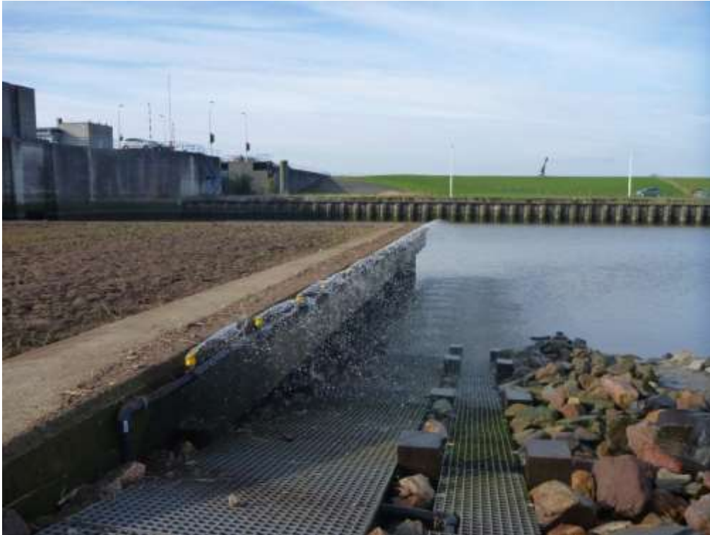
Figure 6.4 Recently constructed elver pass at Nieuwe Statenzijl, Netherlands, employing multiple plunging flow outlets at the downstream end of the pass to enhance attraction and passage
