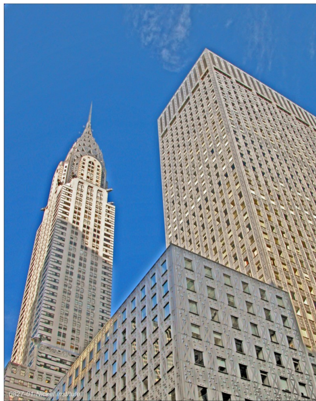
Figure 49: The Socony-Mobil building, after cleaning 40 years of grime from its stainless steel panels. The stainless steel clad peak of the Chrysler building is shown in the background
