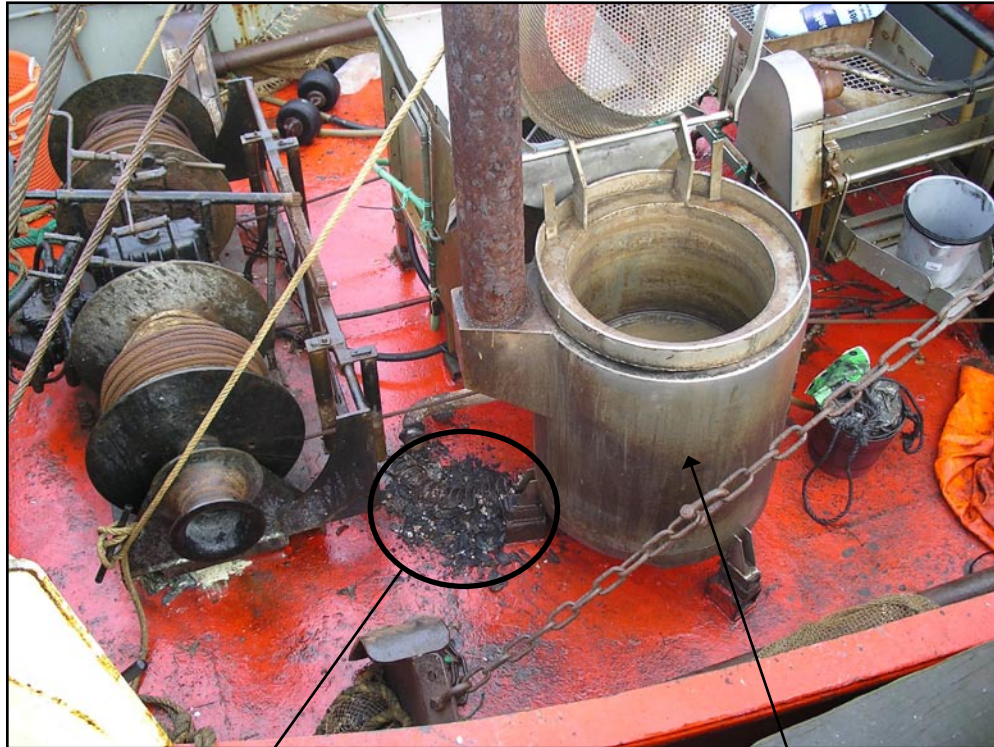
Burnt section of plastic air supply trunking
