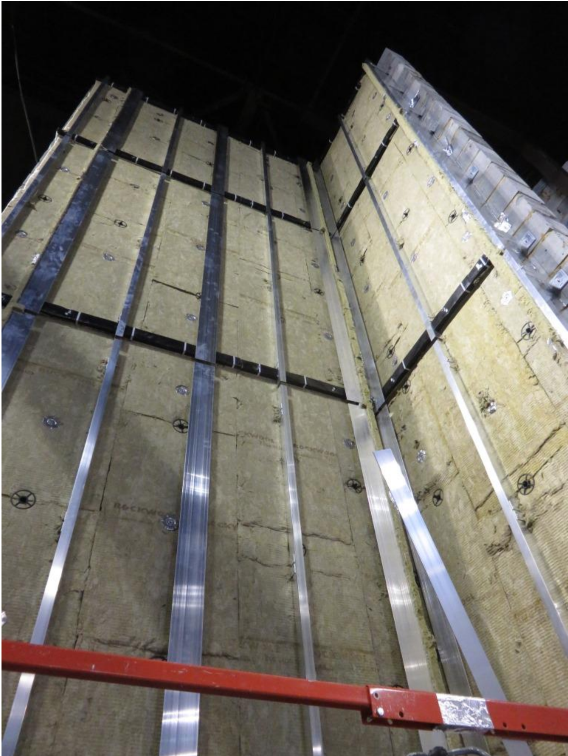
Figure 9. Completed installation of railing substructure visible on main wall.
