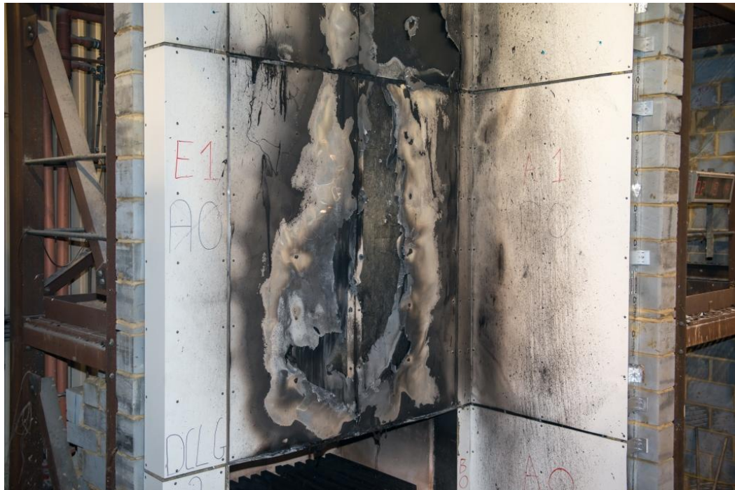
Figure 22. First row ACM panels (directly above combustion chamber).
