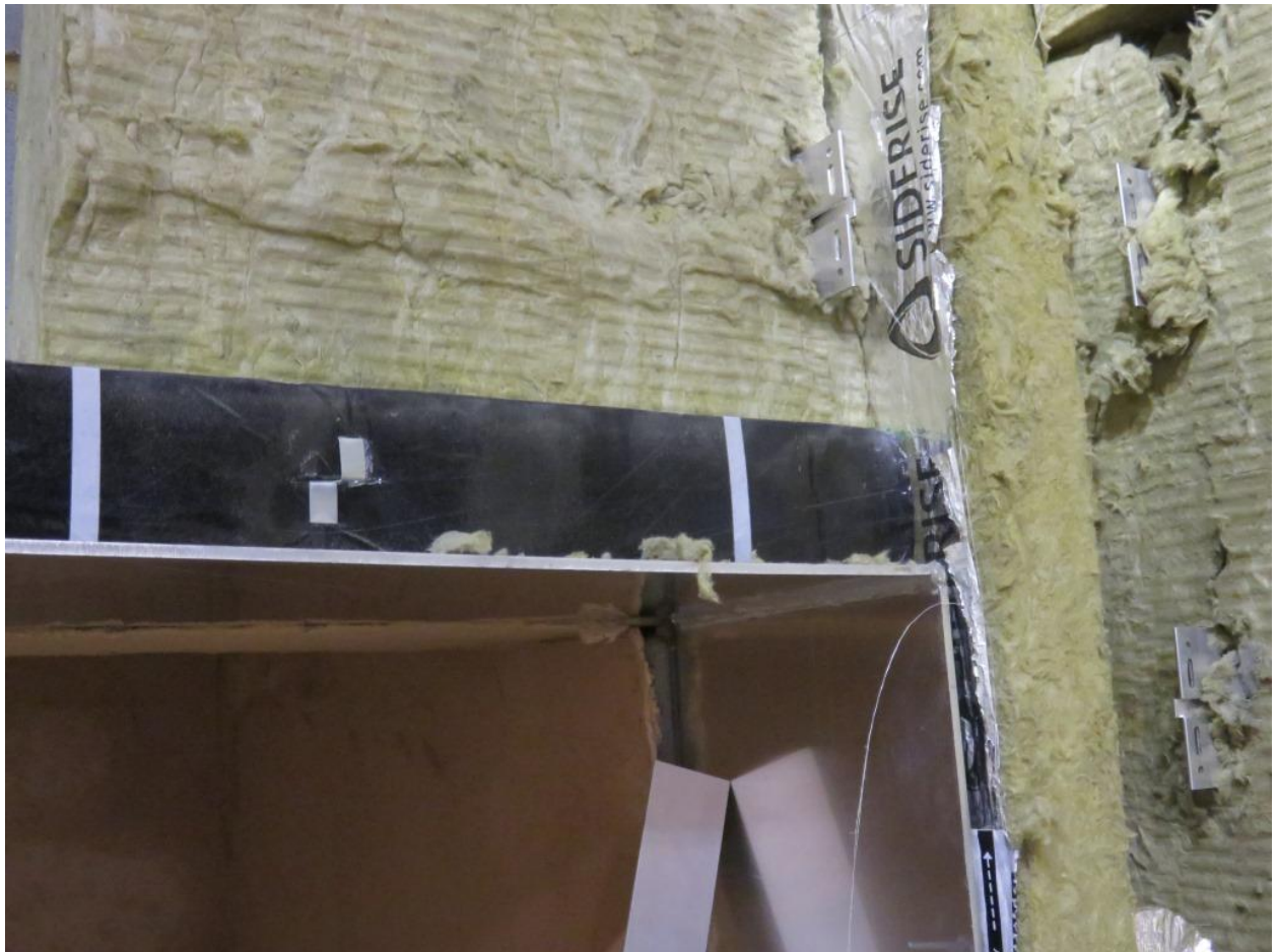
Figure 4. Installed window pod lining combustion chamber.
