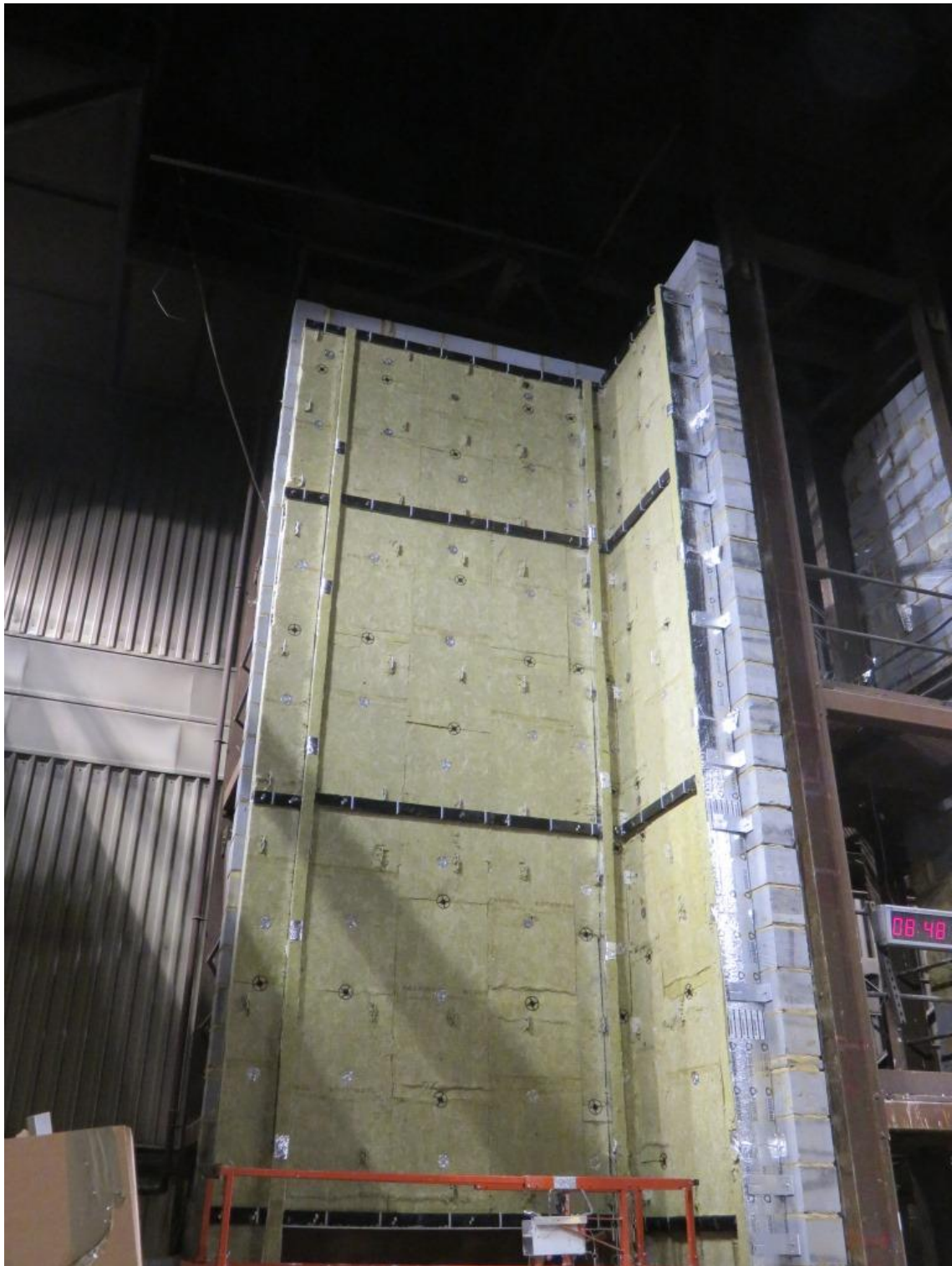
Figure 6. Installed cavity barriers and stone wool insulation.
