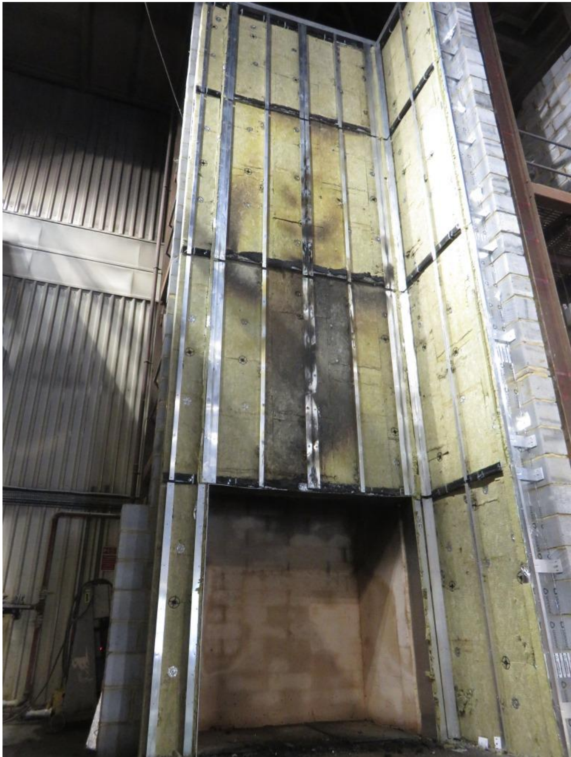
Figure 26. Full height photograph of cladding system following removal of ACM panels.
