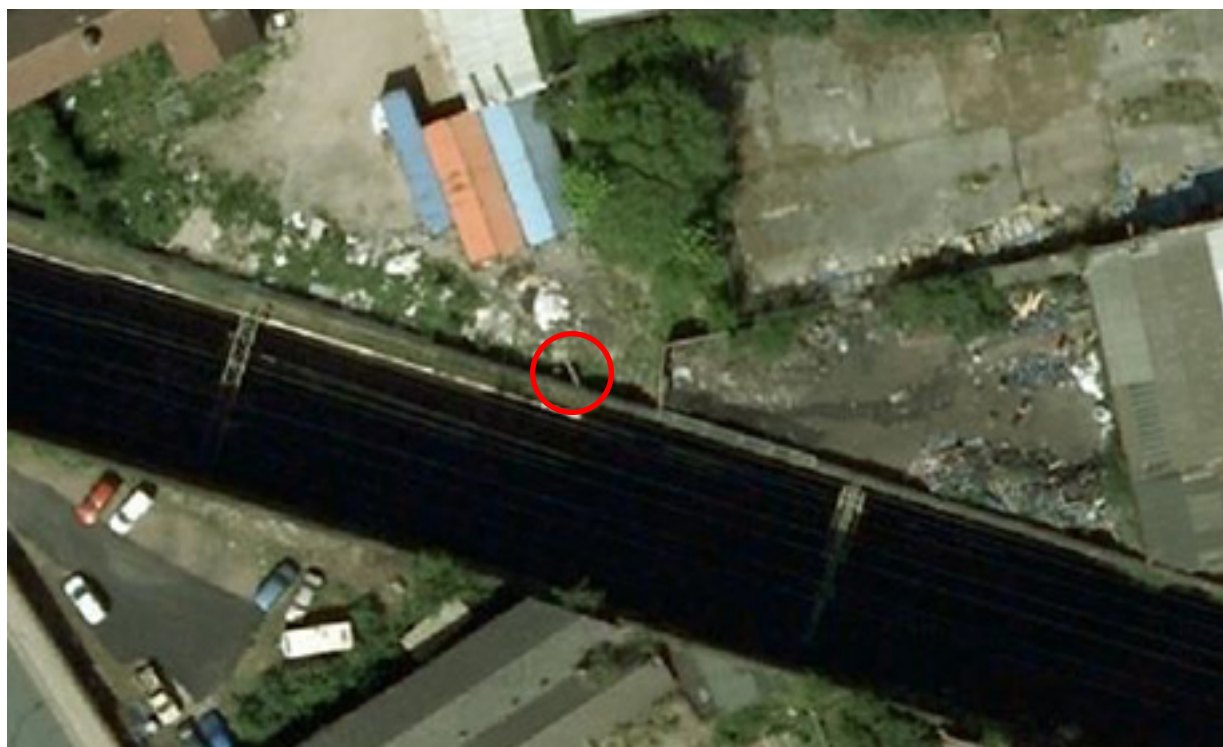
Figure 8: Aerial image of the site taken on 2 September 2005 showing metal storage shelter and shipping containers. The red circle indicates the short section of remaining full height section of the concrete terrace wall (courtesy of Getmapping PLC).
