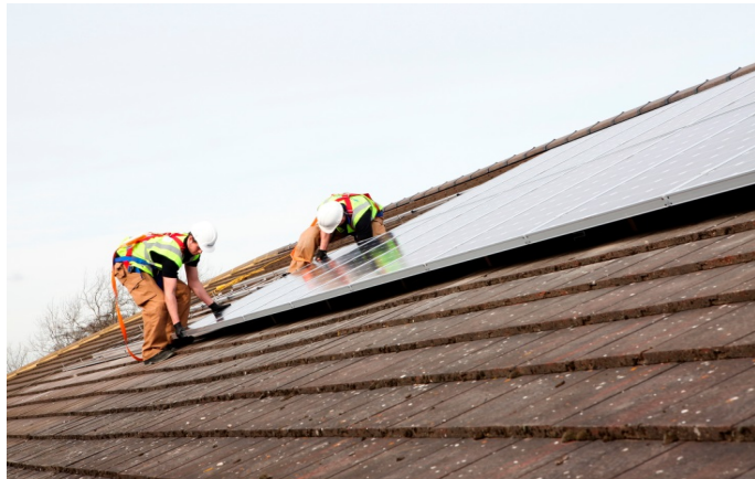
Picture 3. - Installing PV Solar Panels
