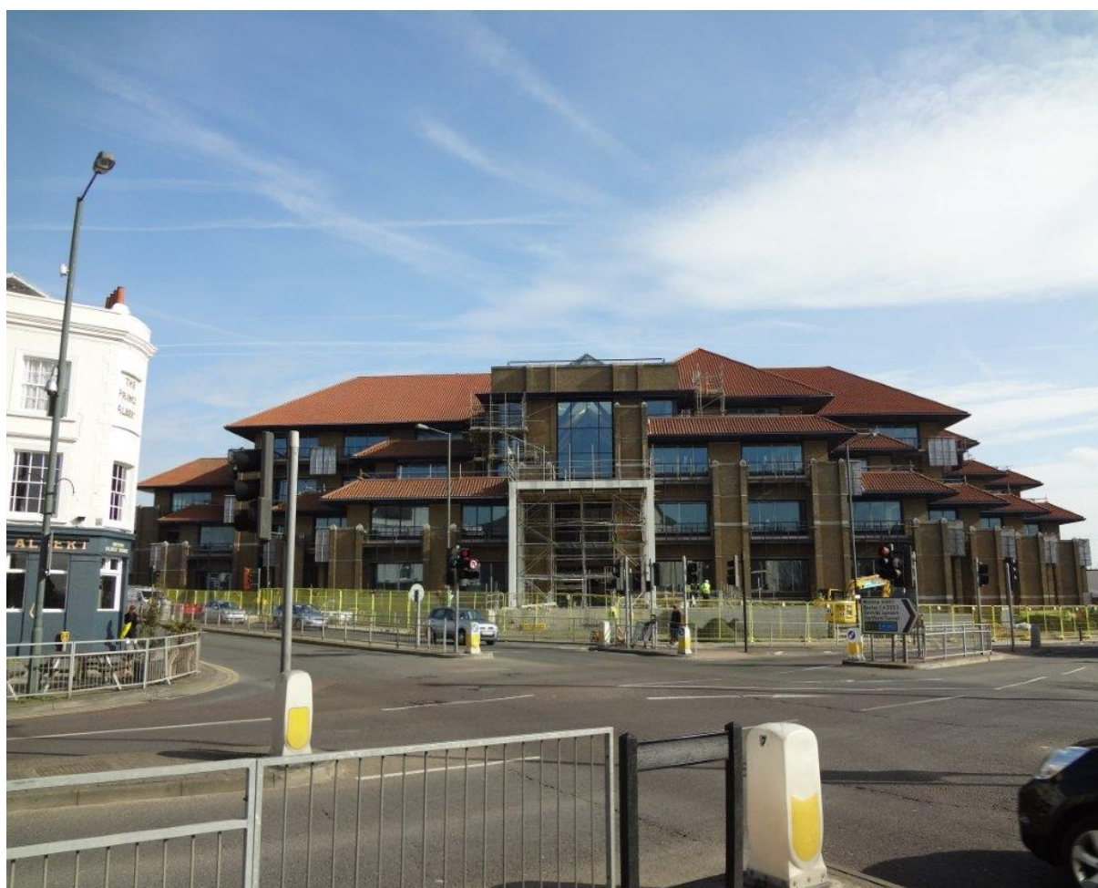
Picture 4. - Conversion of a former bank building to council offices in Bexley
