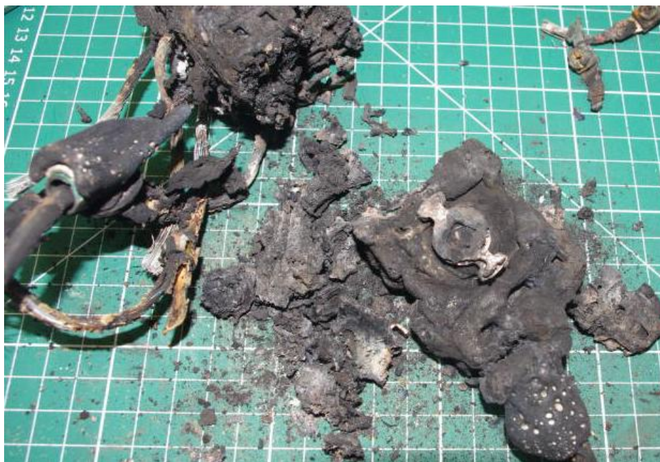
Figure 4: Remains of a DC isolator being disassembled and inspected in the laboratory (Photo courtesy of Fire Investigations (UK) LLP)
