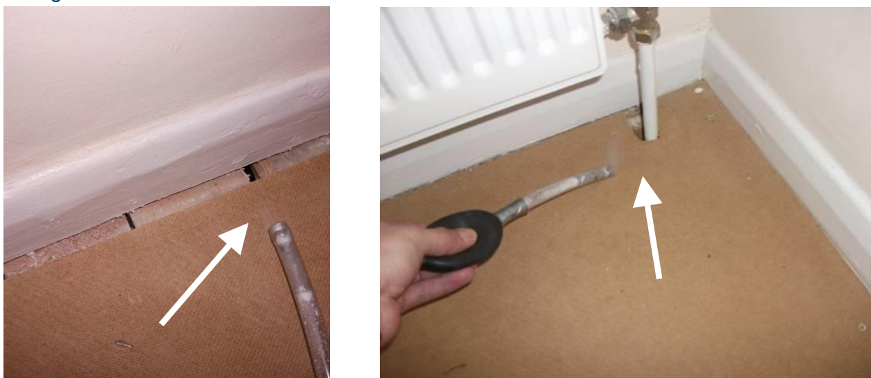
Figure 5: Post-refurbishment air leakage audit of floors with smoke pencil
