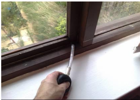
Figure 51: Smoke Pencil testing during air leakage investigations
