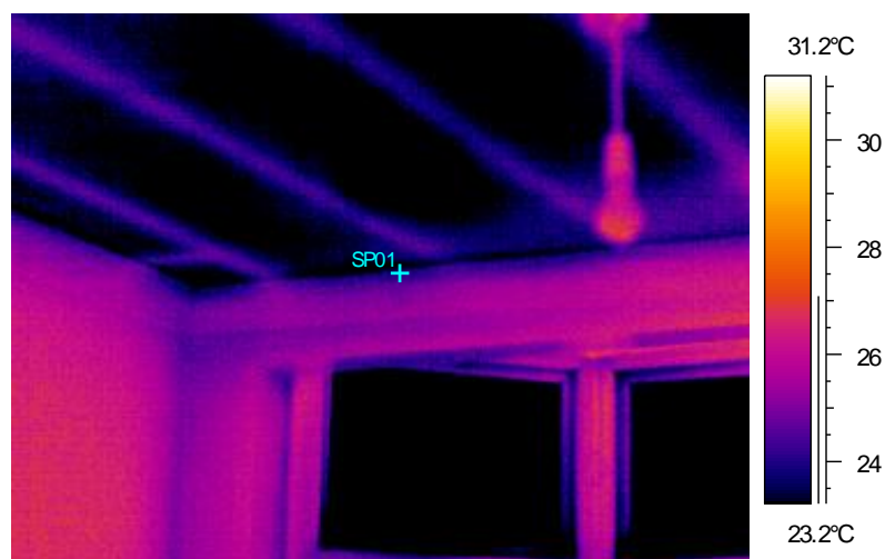
Figure 12: Thermal image of cold ceiling
