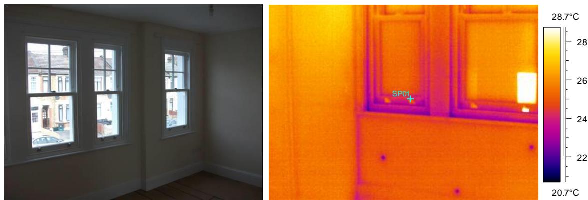
Figure 15: Thermal image of sash windows
