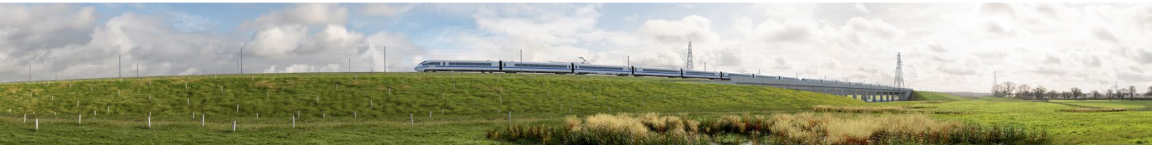
View from Gonsley Green Farm looking towards the proposed Chorlton South embankment and the Blakenhall viaduct (year 1 of operation)
