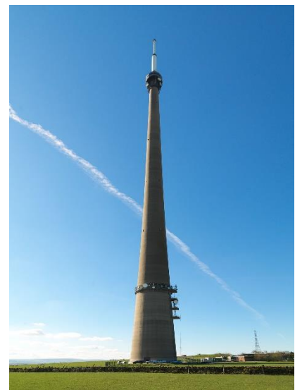
New transmitter (photo Arqiva)
