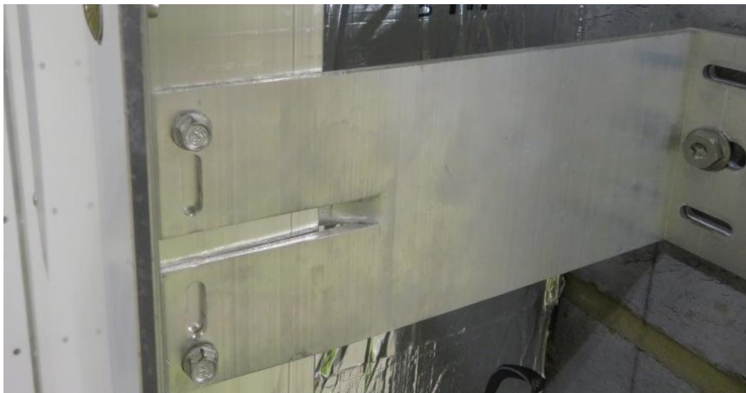
Figure 7. Example of aluminium rail fixed to 'L' bracket through fixed holes.
