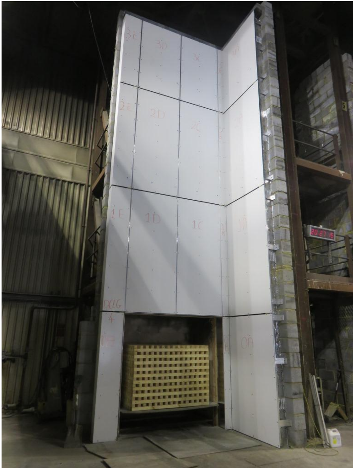
Figure 11. Completed installation prior to test.
