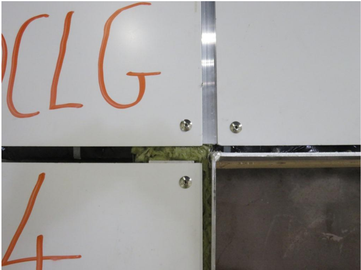
Figure 10. Detail at corner of combustion chamber opening. Panels riveted in place and nominal 20mm vertical gap left for ventilation purposes.
