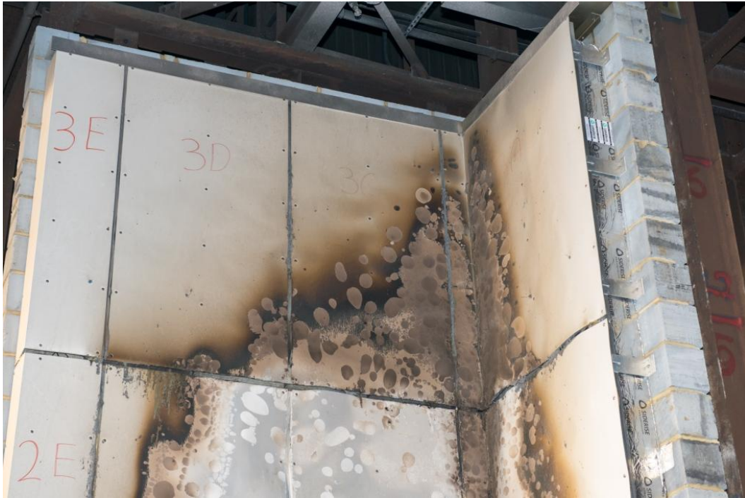
Figure 25. Third row ACM panels (approximately 4600mm-6500mm above combustion chamber).
