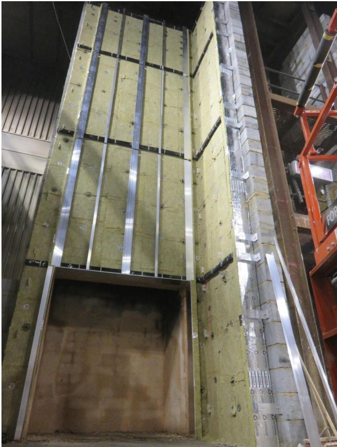
Figure 8. Installation of railing substructure visible on main wall.
