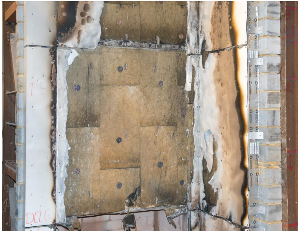
Figure 23. First row ACM panels (directly above combustion chamber).
