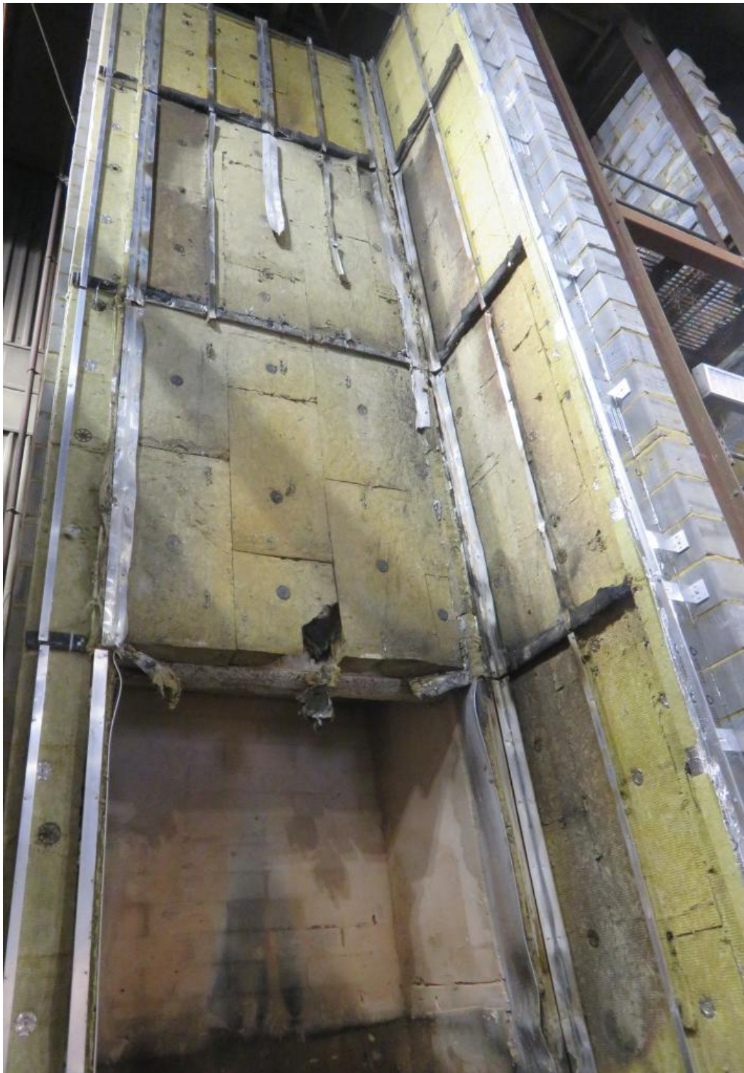
Figure 29. Full height photograph of cladding system following removal of ACM panels.
