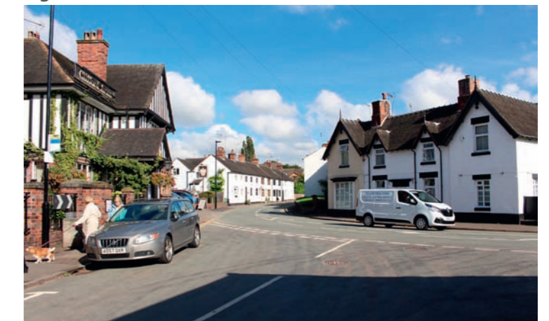
Figure 3: Main Road from Trent Lane
