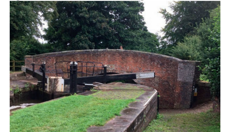
Figure 2: Grade II listed Hoomill Bridge Number 76
