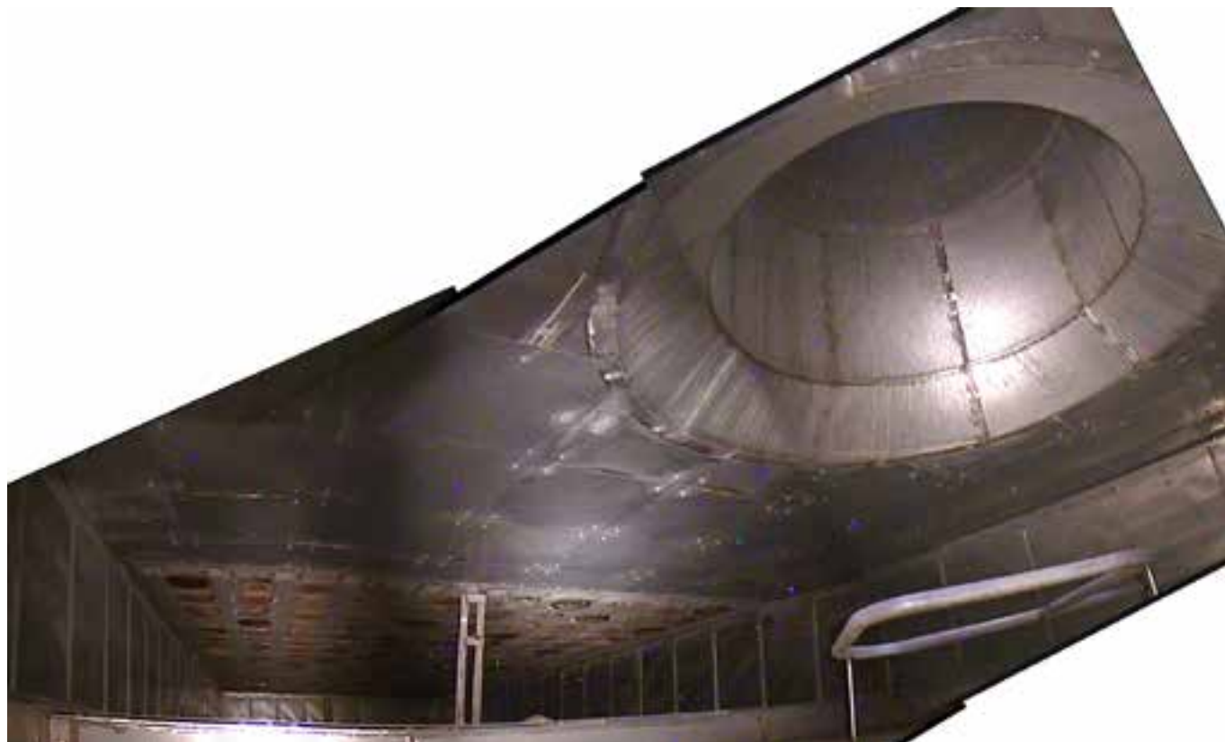
Merged picture of the upper plenum of a storage vault
