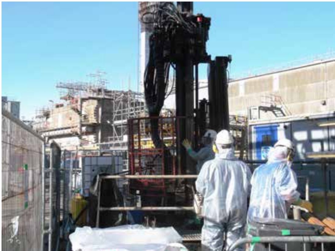
Drilling rig, typical of what would be required to establish a borehole array for the potentially viable intervention technologies
