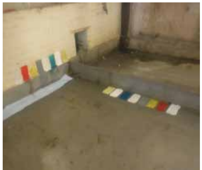
Active Trials in FGMSF, coatings on the left are on painted brickwork on the vertical plain, coatings on the right on stainless steel on the horizontal plain
