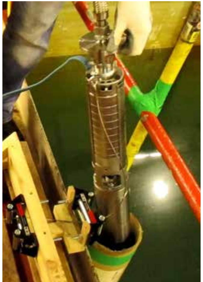
Pump connected to hose, taken during testing of system deployment
