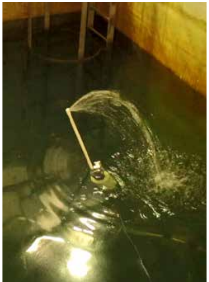
System pumping water in test pond
