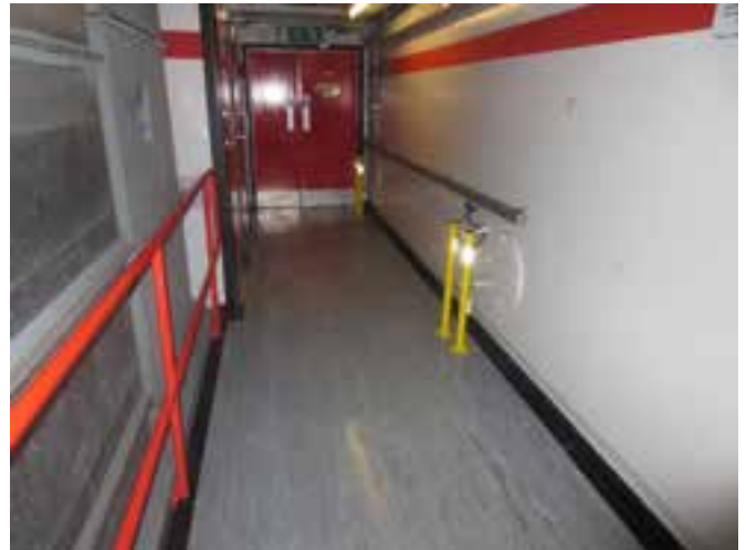
Debris Removal Hatch – access corridor
