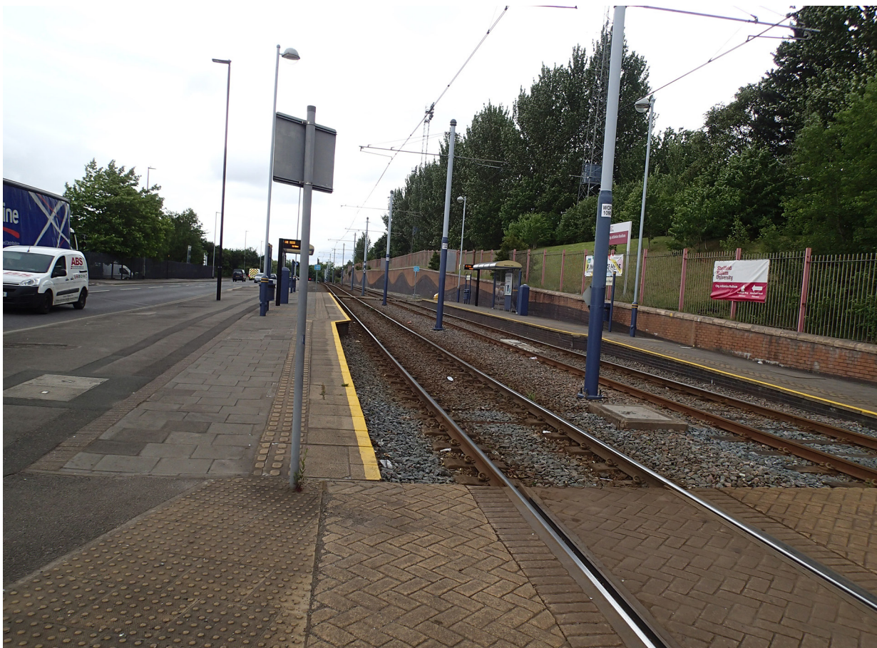
Figure 9: The position of the posts between the tracks through the tram stop
