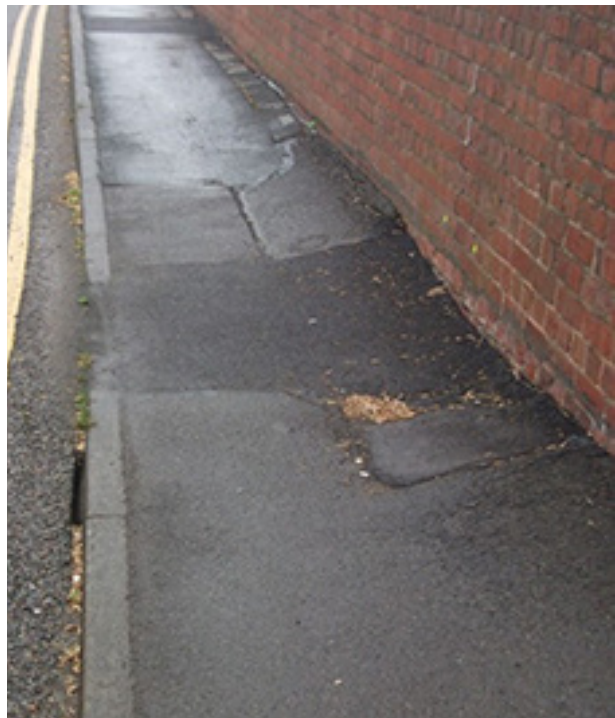
Figure 6f: May 2016 - close-up of area of subsidence (image courtesy of Leicestershire County Council)
