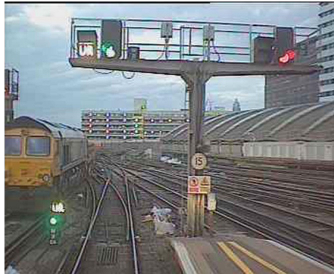
Figure 5: View from the train's forward facing CCTV of the green signal and 'UR' (Up Main Relief) route indication, duplicated at high and low levels, at the departure end of platform 11
