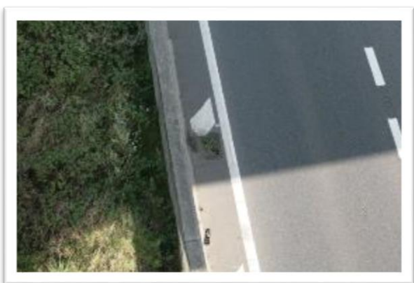
Figure 5-4 The A2 as seen from the Wood Lane overbridge, illustrating a partially blocked highway drain on the eastbound carriageway (left), and silt build-up adjacent to the central concrete barrier on the westbound carriageway (right)
