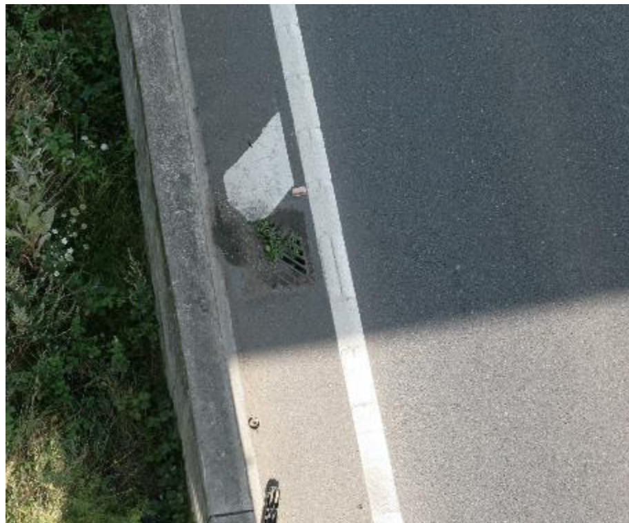
Figure 3-9 Blocked Gully at Wood Lane Overbridge on the A2 Eastbound
