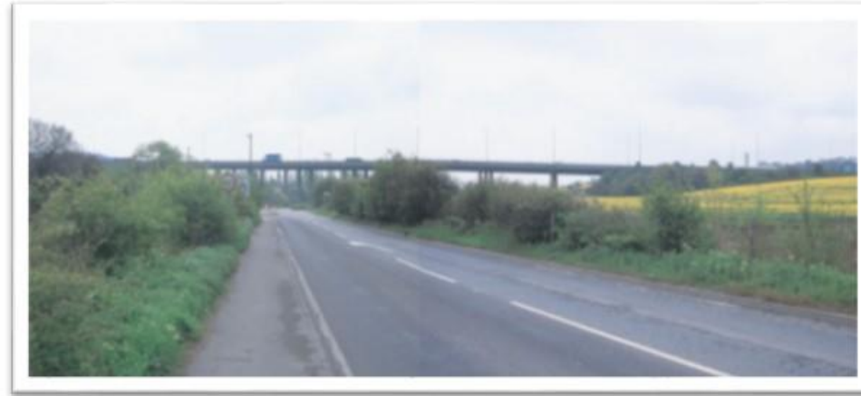
A2/ A282 Dartford Improvement Proof of Evidence for the Public Inquiry, Photograph 2 (c.2004)
