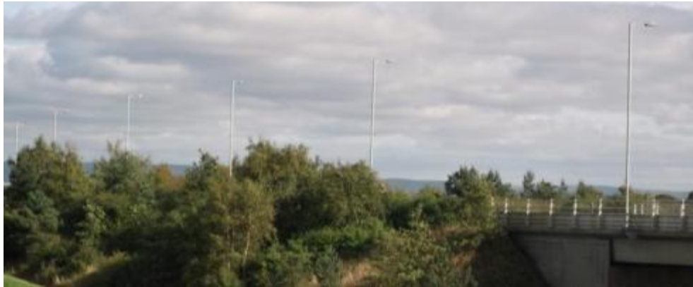
Figure 5.17 – Eastern approach from Gatenby – lighting columns
