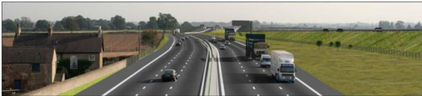
View from Gatenby Overbridge towards the A1 in the year of opening (Year 0).
