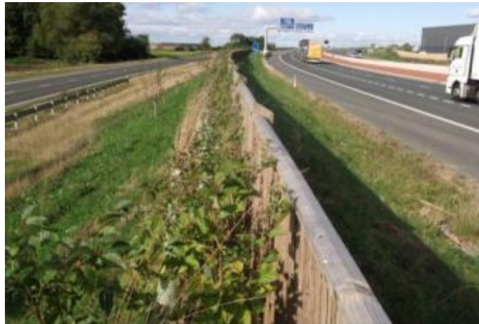
Figure 5.12 – Combinations of earth mounding and anti-glare fencing
