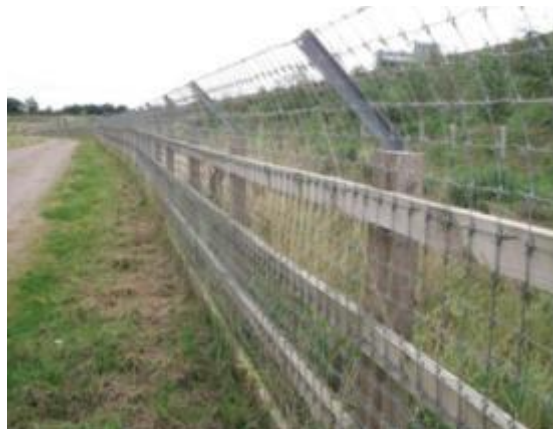
Figure 5.21 – Otter fencing at Bedale Beck North pond
