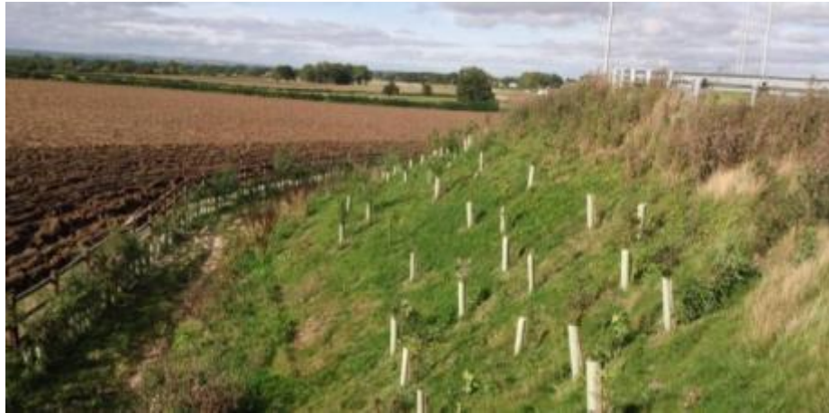
Figure 5.11 – Strengthened slope west of Gatenby Overbridge
