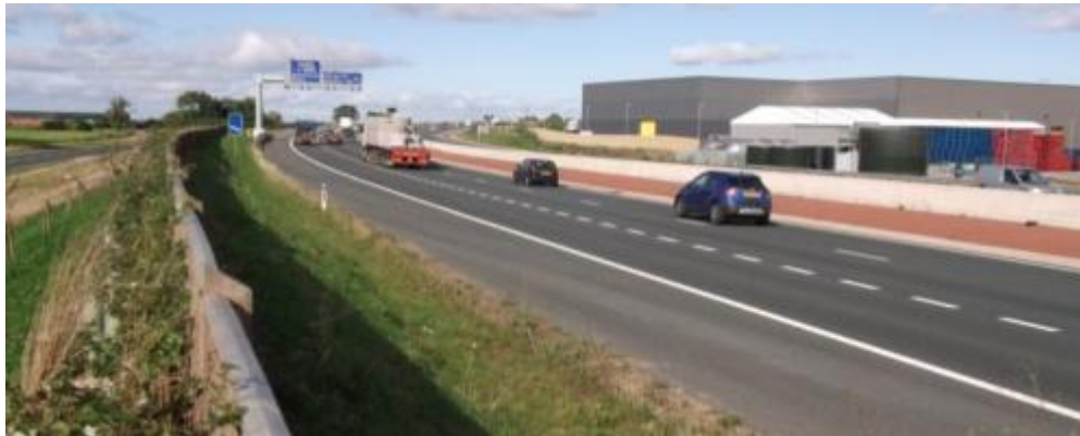
Figure 5.4 – Industrial development along the A1(M) near the Northalleton/Bedale junction
