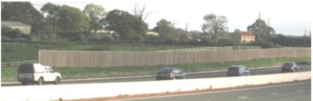
Figure 5.3 – Noise barrier at Burneston Grange
