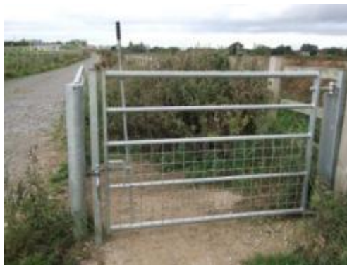
Figure 5.37 – Access gate for horse riders in the foreground, bridleway in the background running adjacent to the A1(M)
