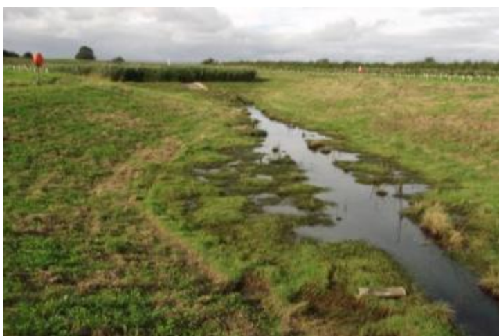
Figure 5.31 – Hergill balancing pond showing area (in foreground) provided to accommodate any overflow in periods of heavy rainfall
