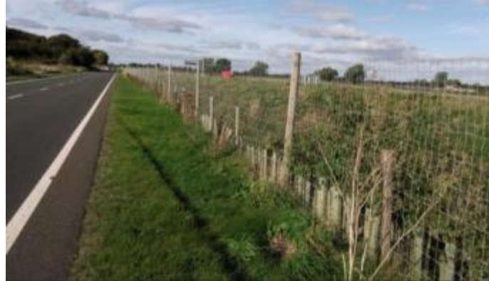
Figure 5.22 – Deer fencing between the LAR and A1(M)
