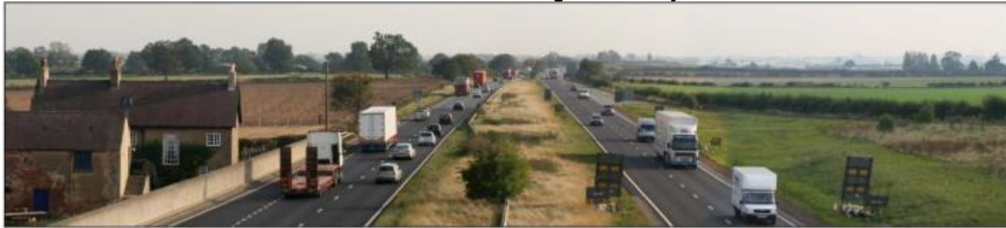
Existing view from Gatenby Overbridge towards the A1.
