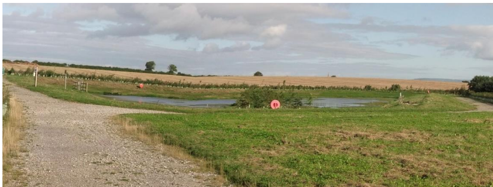
Figure 5.29 – Rainton Balancing Pond
