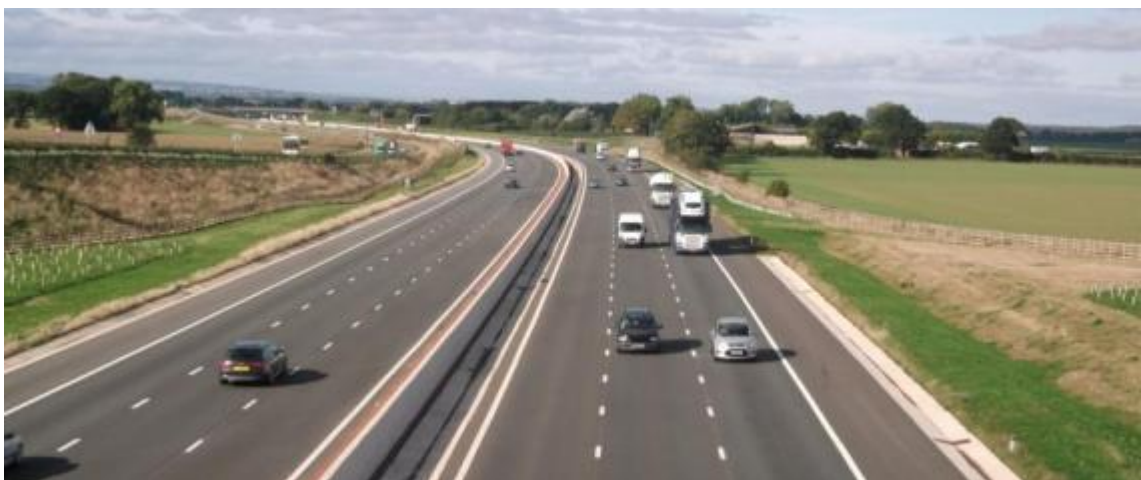
Figure 5.1 – View of the scheme looking north from the Gatenby Overbridge
