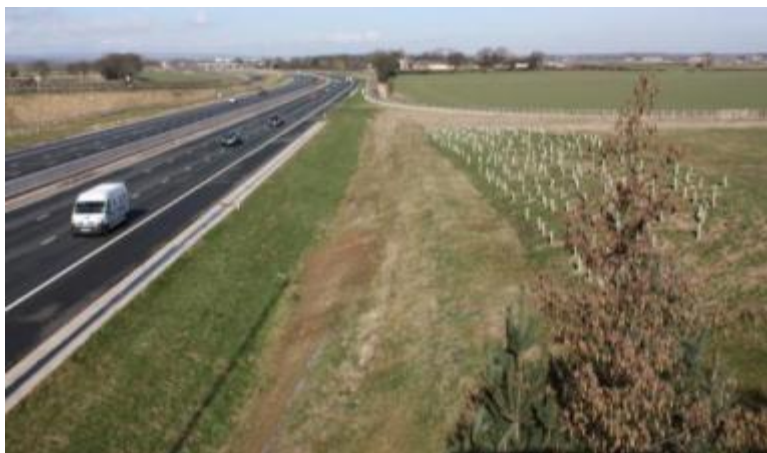
Figure 5.30 – Swale north of Gatenby Overbridge
