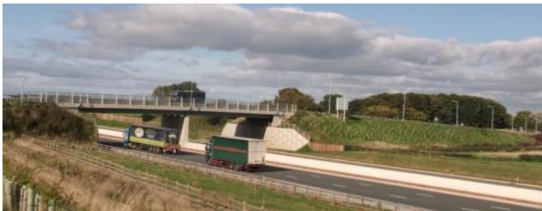
Figure 5.18 – Londonderry Overbridge, including the eastern approach showing introduced lighting columns and mitigation planting
