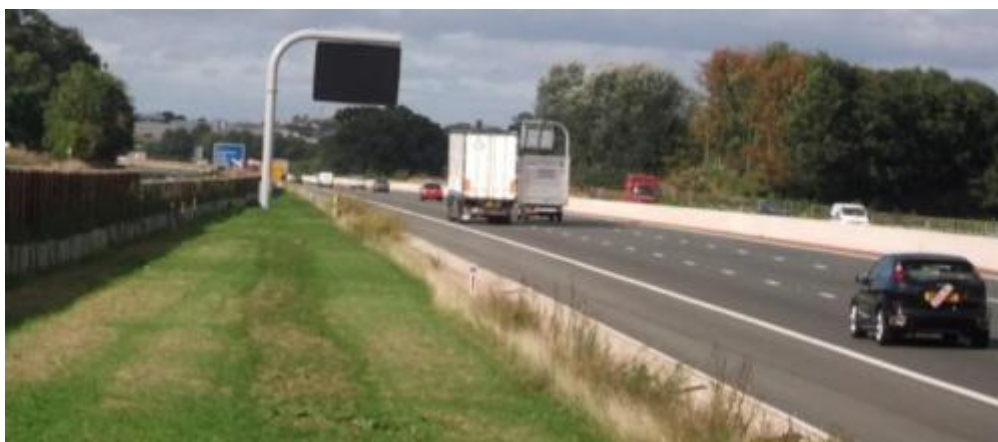
Figure 5.10 – Grass cutting for visibility splays and adjacent to the road have not been undertaken by the Managing Agent
