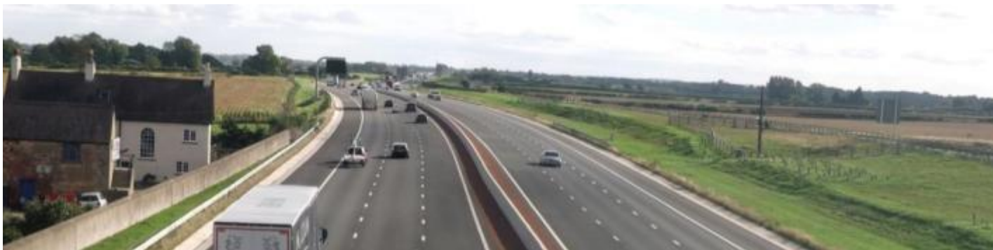
View from Gatenby Overbridge towards the A1(M) one year after opening (photograph taken in October 2013)
