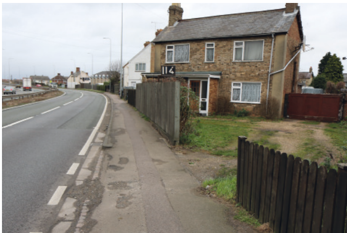
Photograph 8 - Sandy - Black Cat Roundabout. Poor townscape, poor quality footways and hazardous vehicular accesses.
