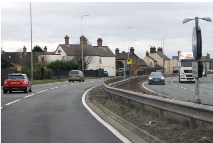
Photograph 4: A421-Sandy, non-motorway section, dual carriageway through established communities
