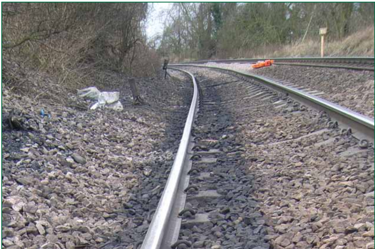
Figure 3: General view of the curve at Santon close to milepost 26
