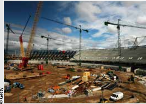
Construction and fitout
