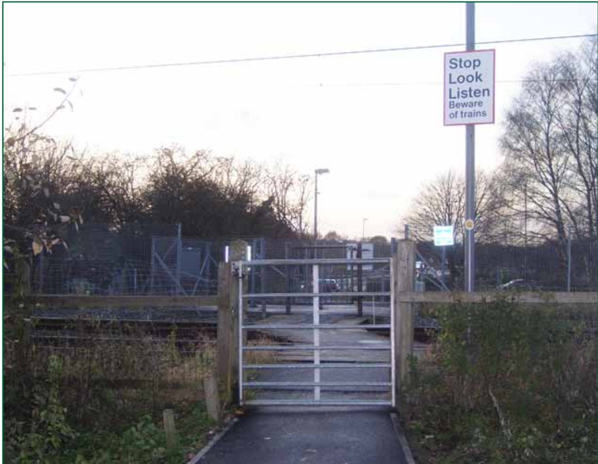
Figure 4: East-side gate from the footpath approach
