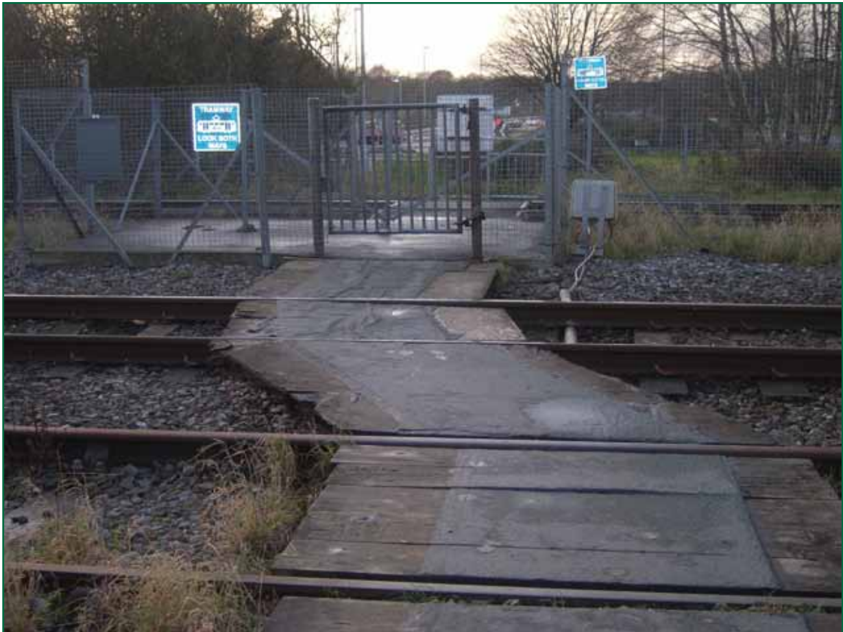
Figure 19: Bayles and Wylies footpath level crossing, showing offset to south
