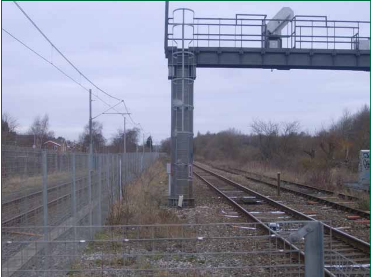
Figure 15: Signal gantry as seen from west-side gate
