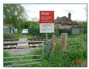
Figure 4: Notices and telephone on the up side at Fairfield crossing
