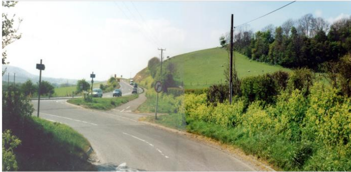
Figure D.13 – View of A27 westward from junction with Ranscombe Lane (pre-construction)
