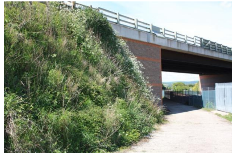
Planting on Railway Bridge abutment
