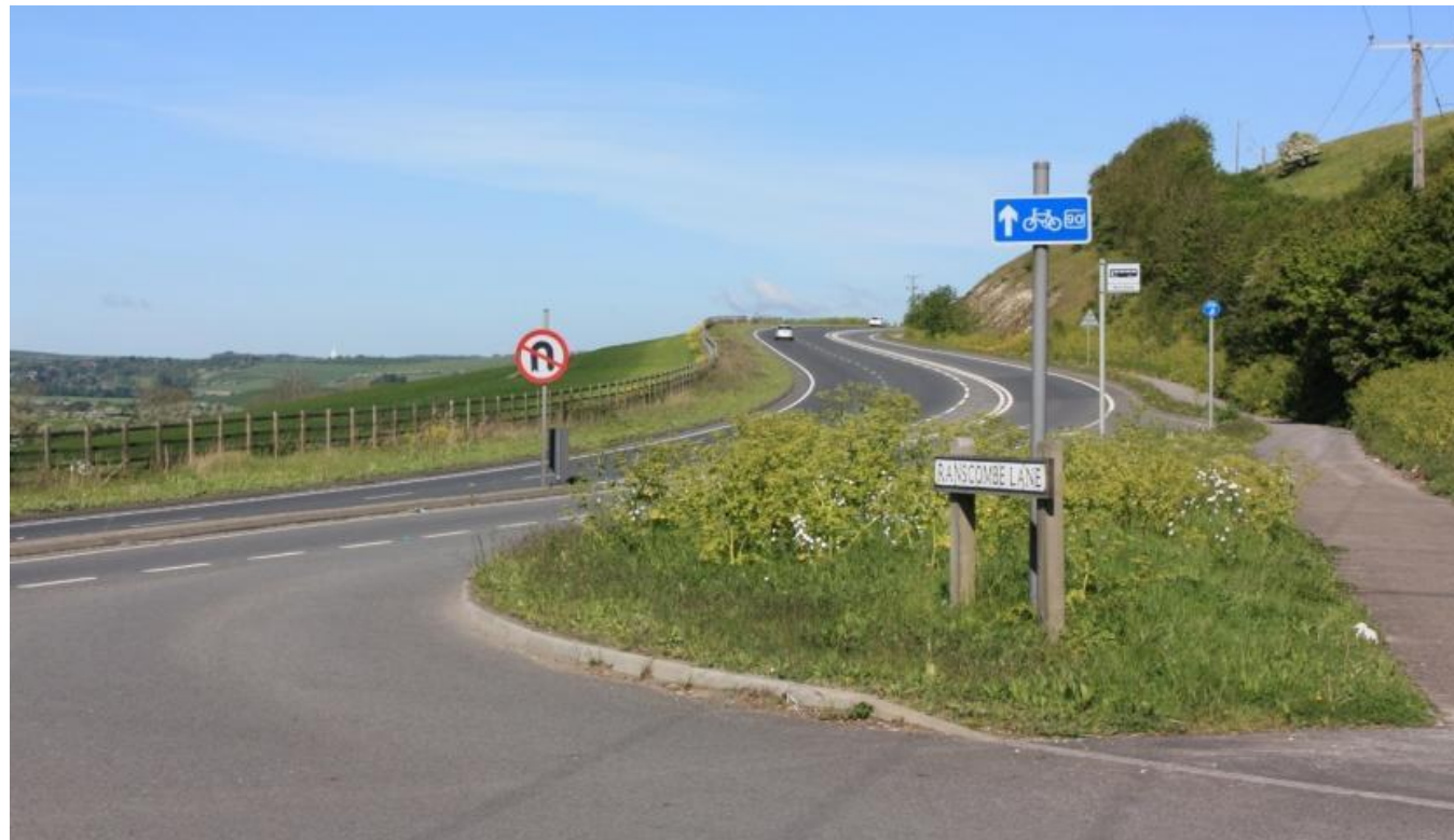
Figure D.15 – View of A27 westward from junction with Ranscombe Lane (Five year after opening)
