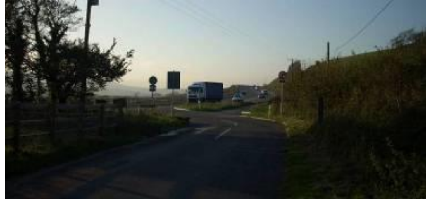
Figure D.14 – View of A27 westward from junction with Ranscombe Lane (one year after opening)
