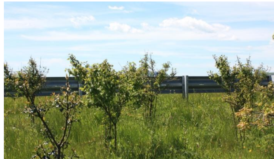
Planting at top of embankment near Railway Bridge
