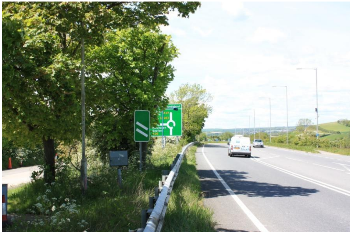
Figure D.18 – View of eastern approach to Beddingham Junction (Five year after opening) showing information signs not visible at OYA
