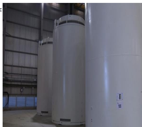
Image of HI-STORM located within Sizewell Dry Fuel Store. HI-STORM will contain spent nuclear fuel when the facility becomes fully operational
