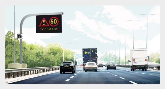
This will involve permanently converting the hard shoulder into a running lane.
