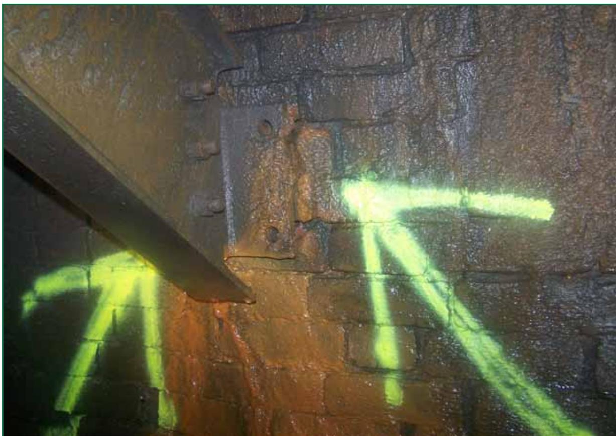
Figures 18 and 19: Missing studs at chainage 34 in November 2008 (photographs courtesy of Network Rail)
