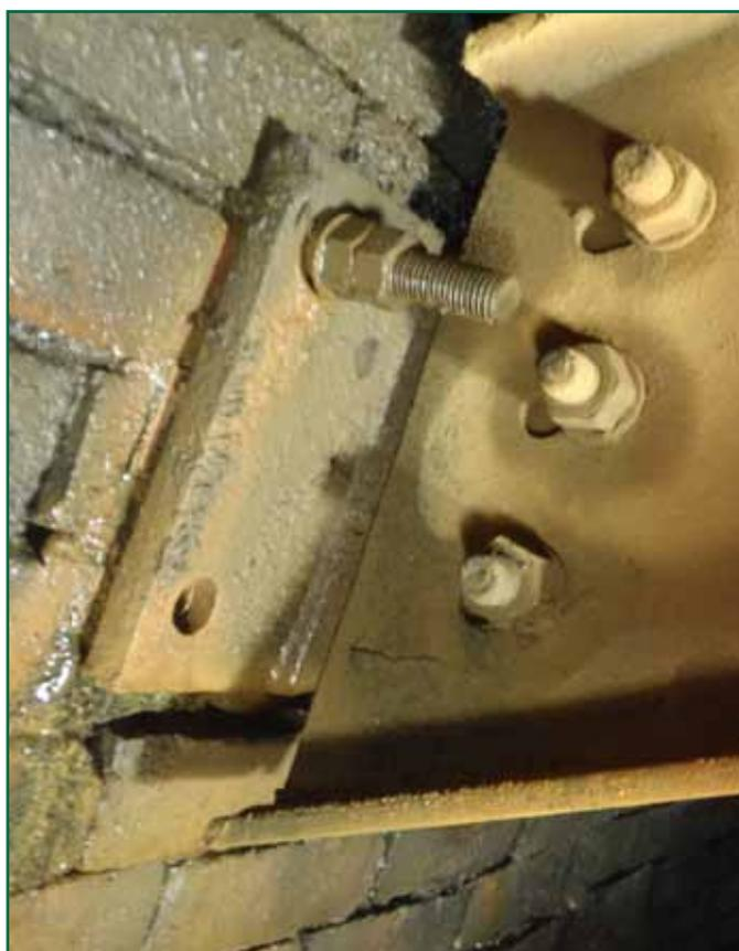
*Figure 11: Bracket with lower stud found missing
