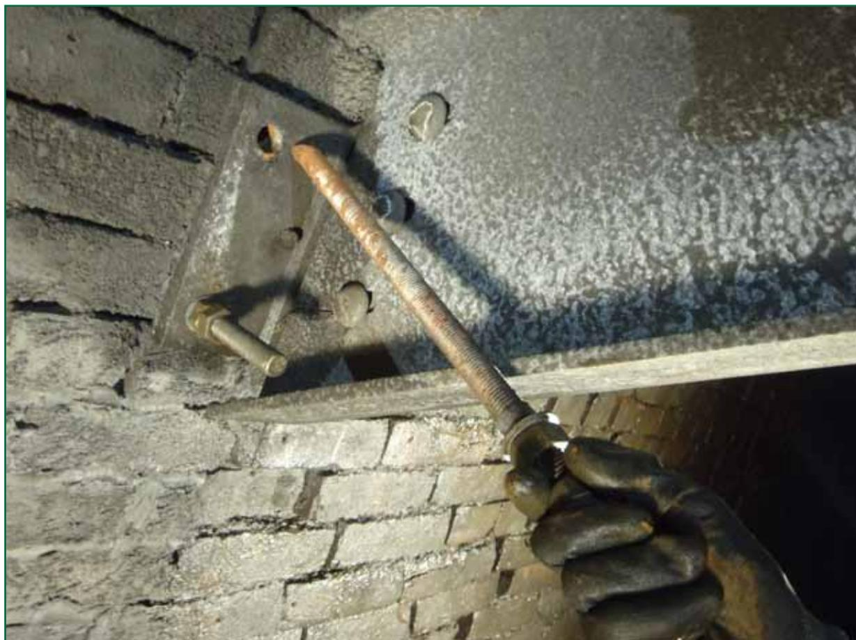
Figure 12: Loose stud outside incident area removed by hand during inspection on 23 September 2011 (photograph courtesy of Amey)
