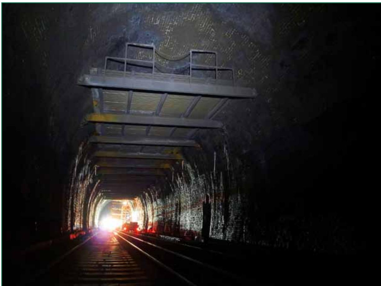
Figure 3: Water catchment tray 5 from north end in February 2012
