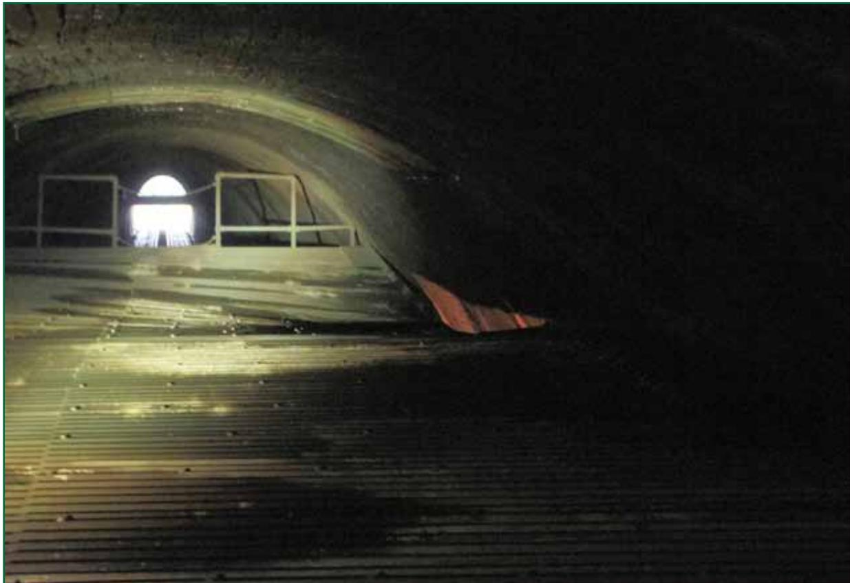
Figure 10: View of deflected structure from above, looking towards the south end of the tunnel, showing the twisted deck on the right-hand side (photograph courtesy of Amey)
