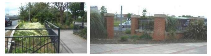
Figure 7-14 Examples where a splash strip was or was not provided at edge of kerb
