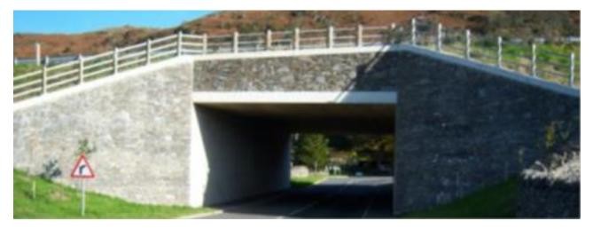
Figure 7-6 Stone faced headwalls at new culvert/mammal tunnel below the A590 High and Low Newton Bypass
